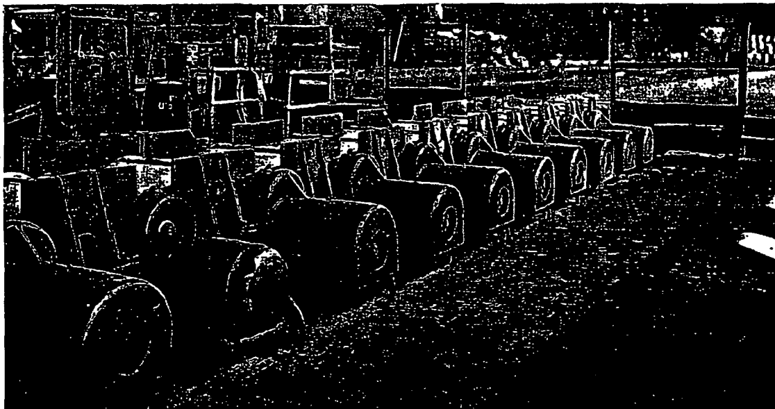
A view of the individual roll drives on runout tables, taken from the finishing stand. 87 motors and 87 rolls comprise this installation.
