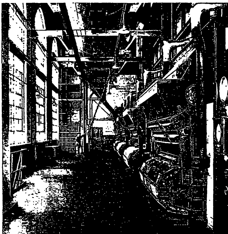
Firing aisle in the boiler room.
