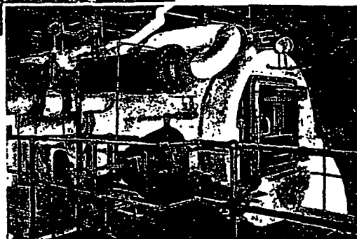
Elliott domestic hot water deaerator installation, which assures corrosionless hot water and freedom from pipe renewals for Indiana University Hospital.
