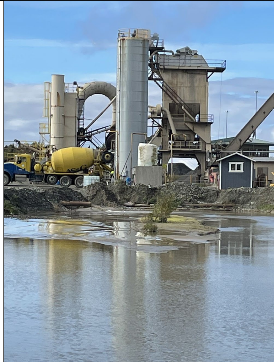
Picture 8: Anchorage Sand & Gravel Pond and Ready Mix Truck at Granite Construction Ready Mix Plant
