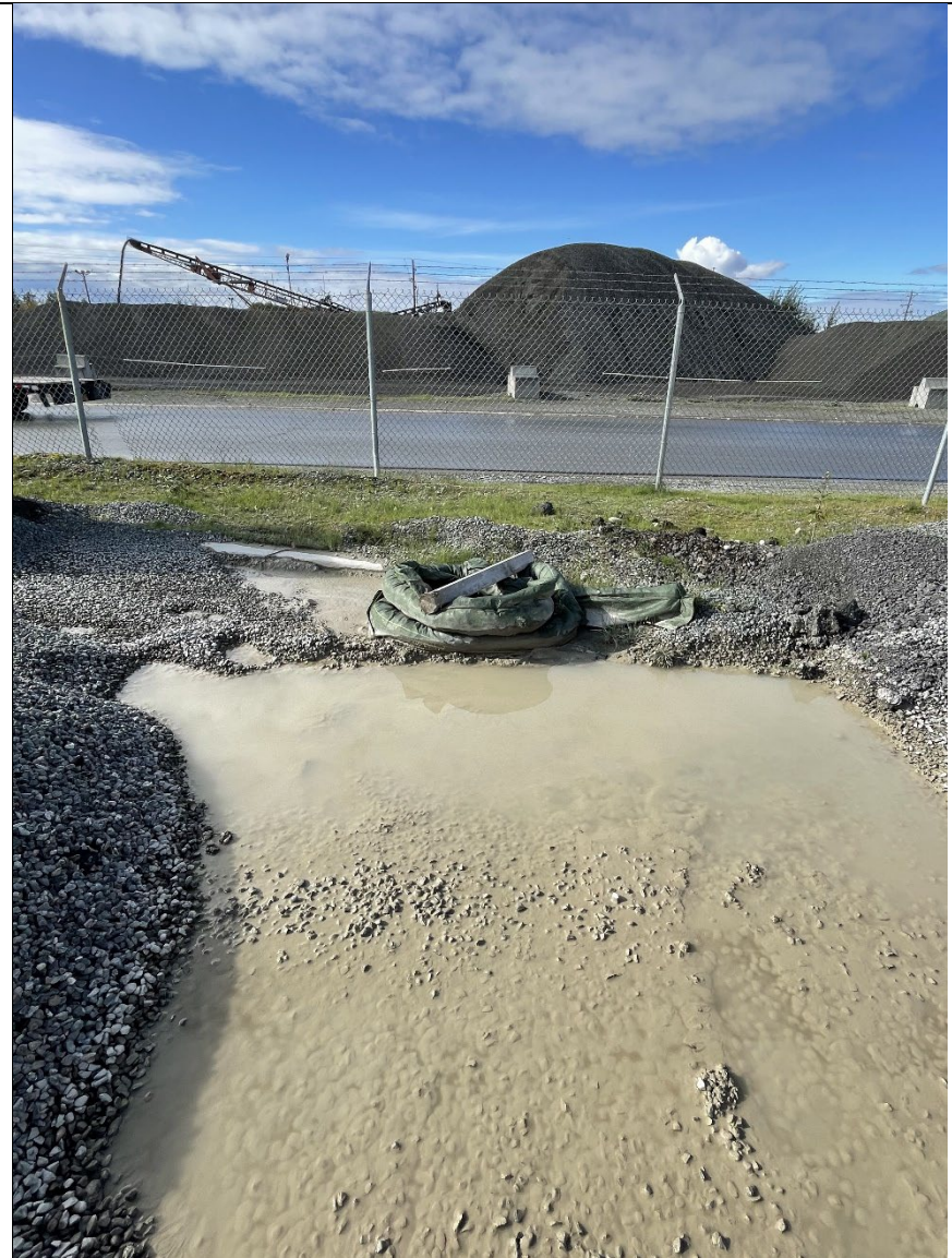
Picture 14: Stormwater Control
