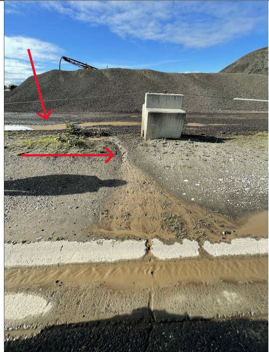
Picture 20: Discharge from RAP Processing Area
