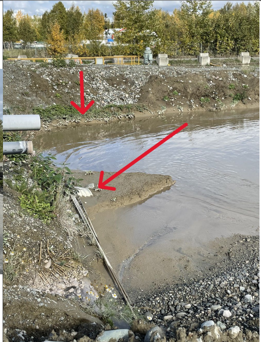
Picture 12: Onsite Pond Mudline and Buried Pipe
