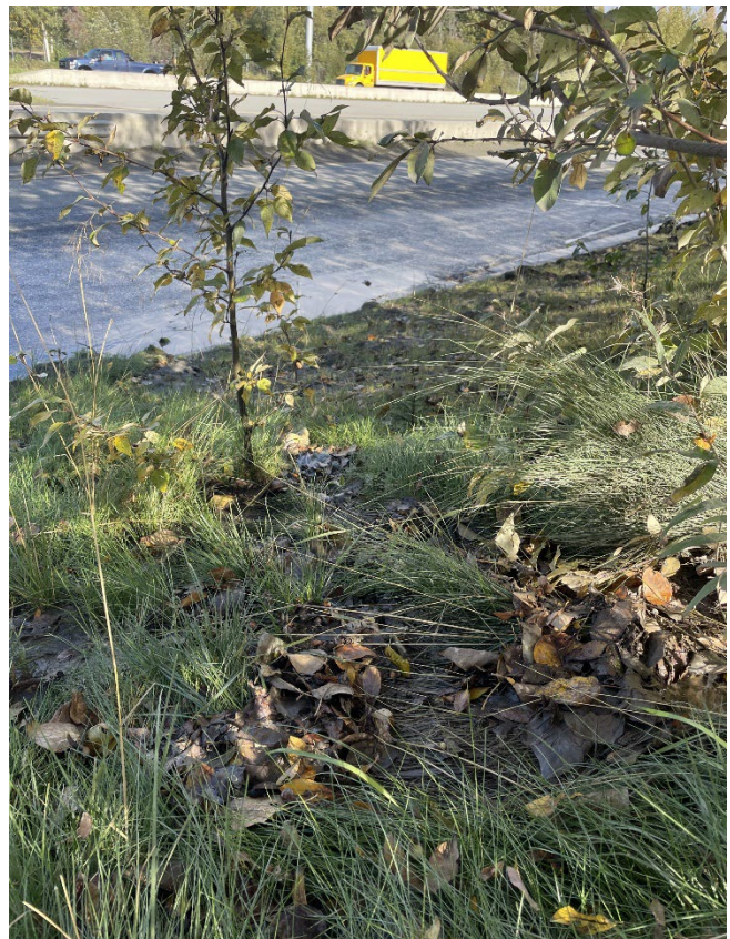
Figure 5: Path of Discharge through Cut, Muddy Grass/Leaves
