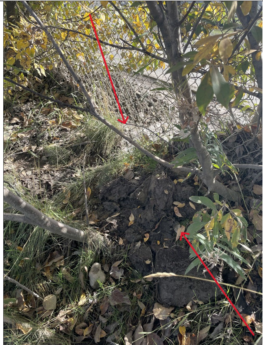
Picture 28: Apparent Removal of Mud from Discharge Location along Northern Facility Road
