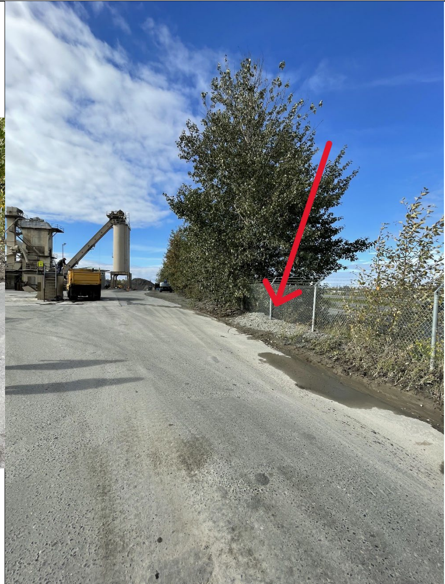
Picture 10: Gravel Installation
