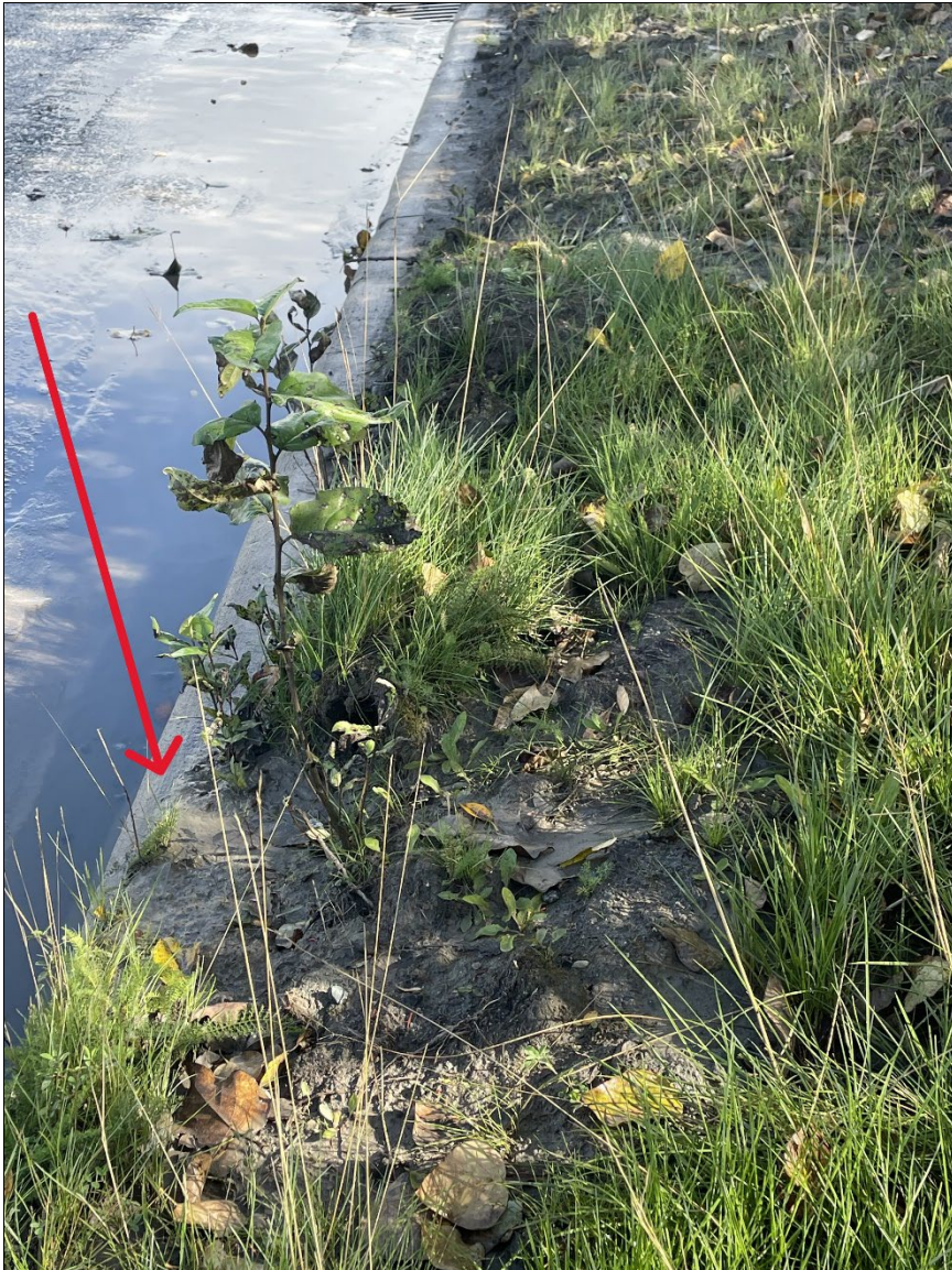
Picture 31: Discharge and Sediment from Northern Facility Road
