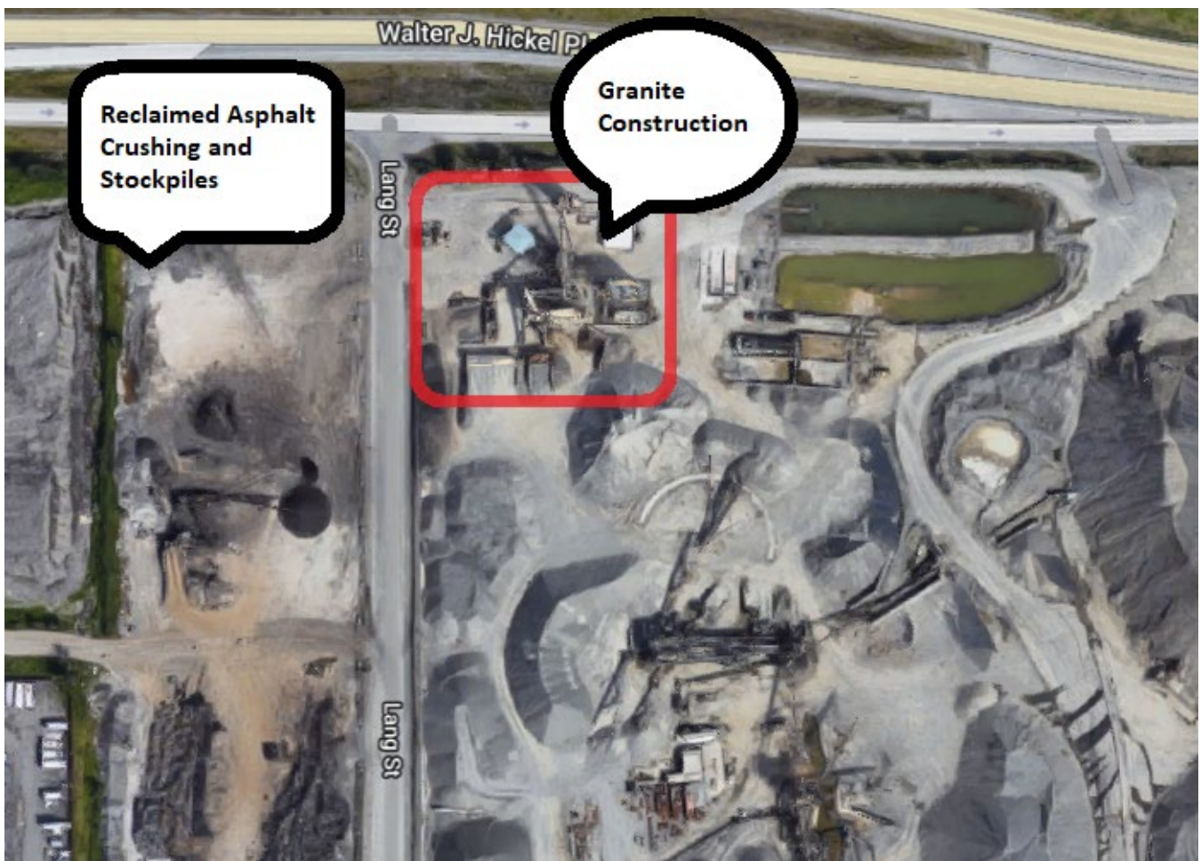
Figure 10: Granite Construction / Reclaimed Asphalt Crushing & Stockpiles
