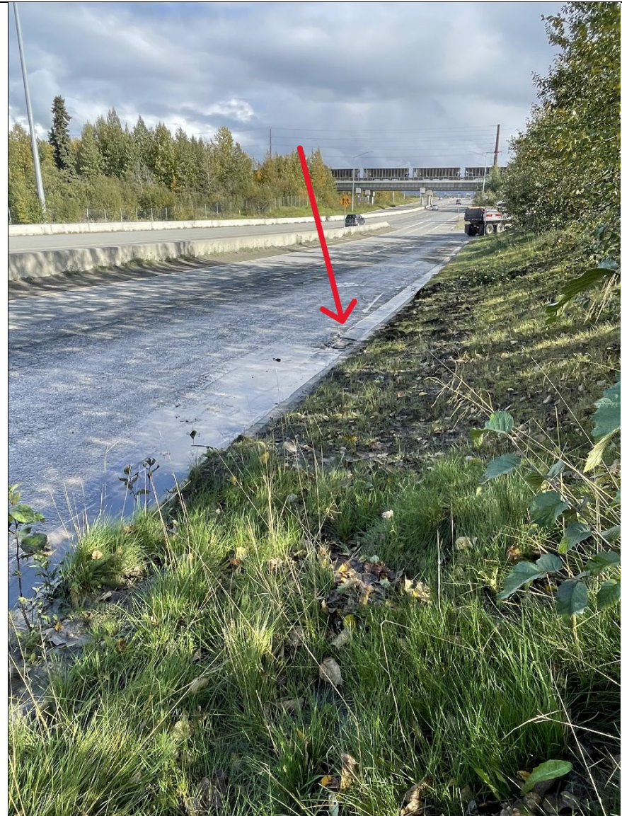
Picture 30: Storm Drain in Gilman Pkwy Gutter
