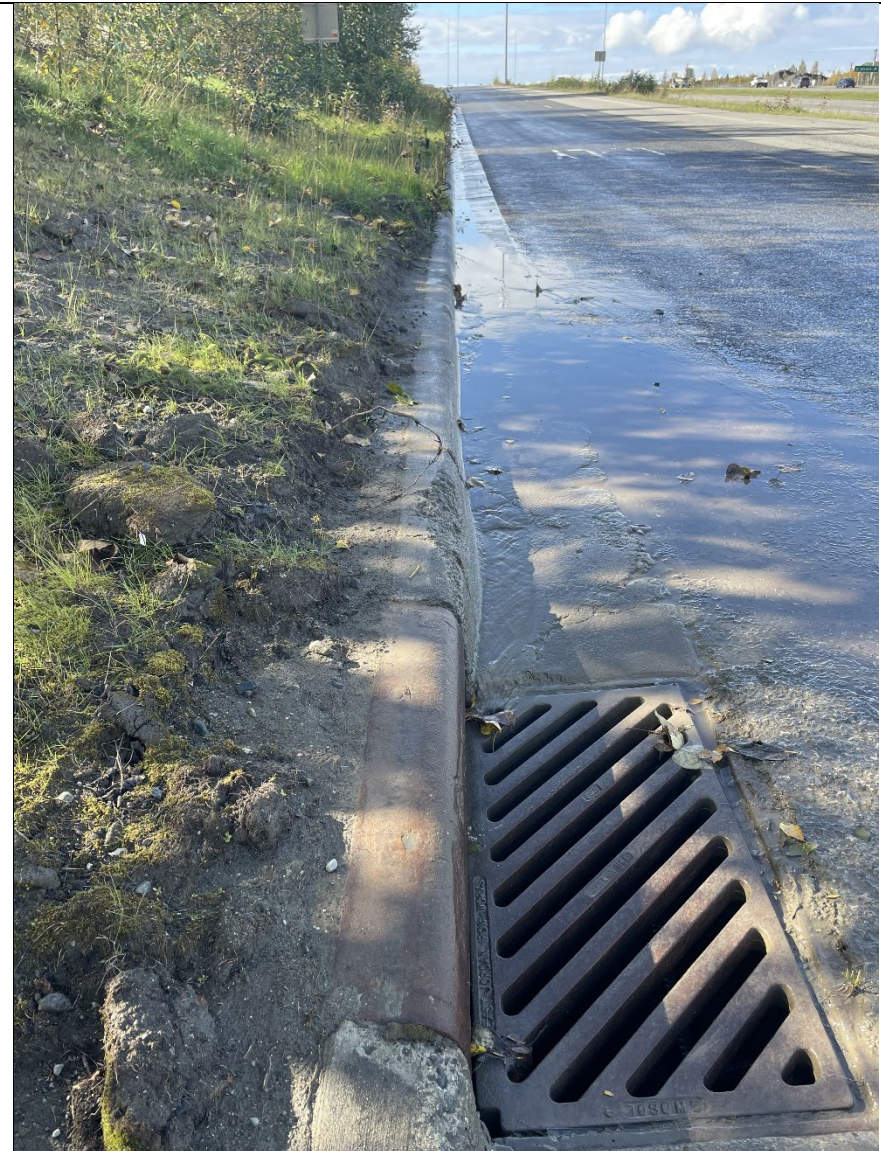
Picture 34: Storm Drain in Gilman Pkwy
