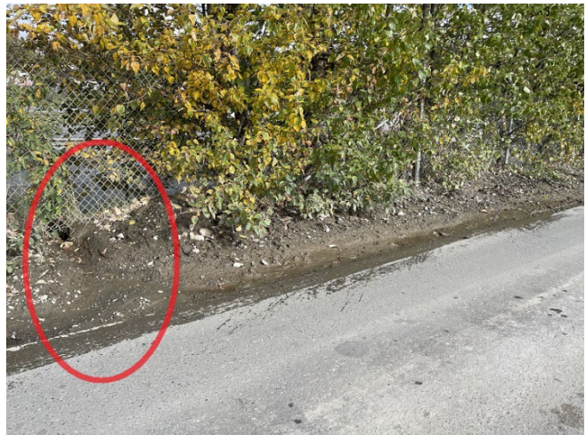
Figure 3: Facility Road Along Northern Boundary with Cut
