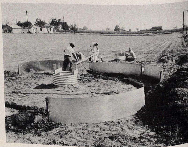
FIGURE 13. Digging trench for dike
