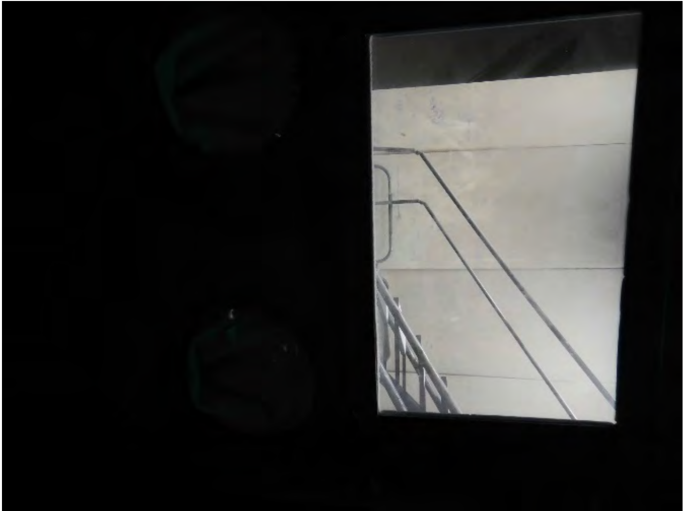
471 – Window on bead blast unit building 282
