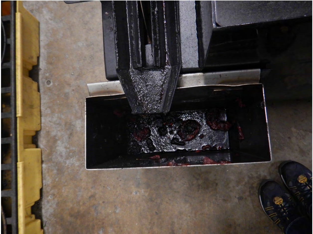
433 – Sludge accumulation from parts washer in building 356
