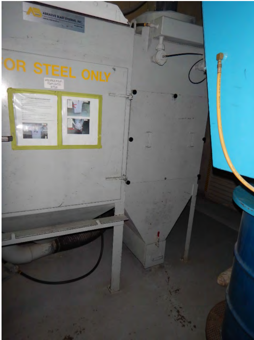
467 – Glass media blast unit building 282
