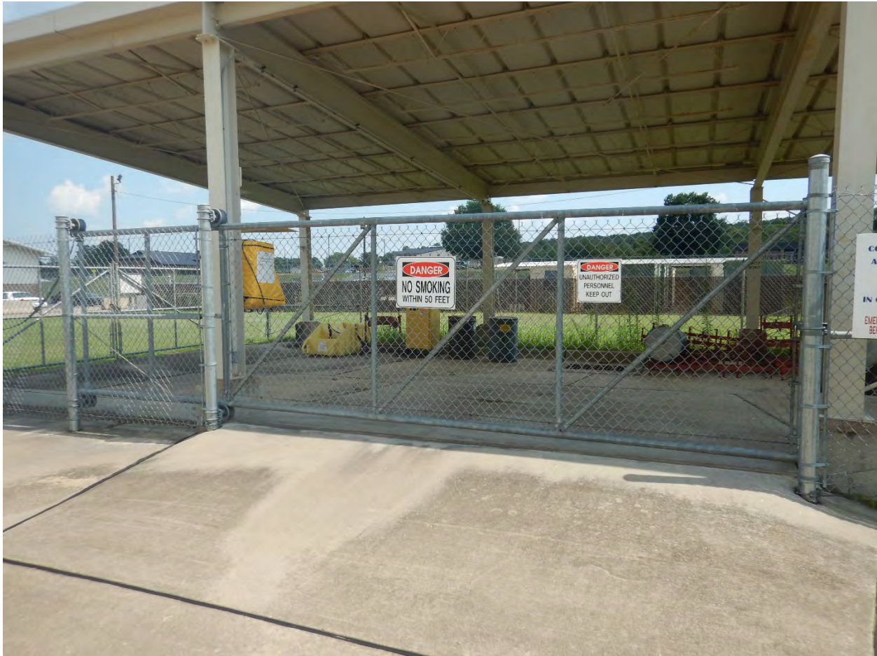
452 – Hazardous waste in 90-day accumulation area outside building 282
