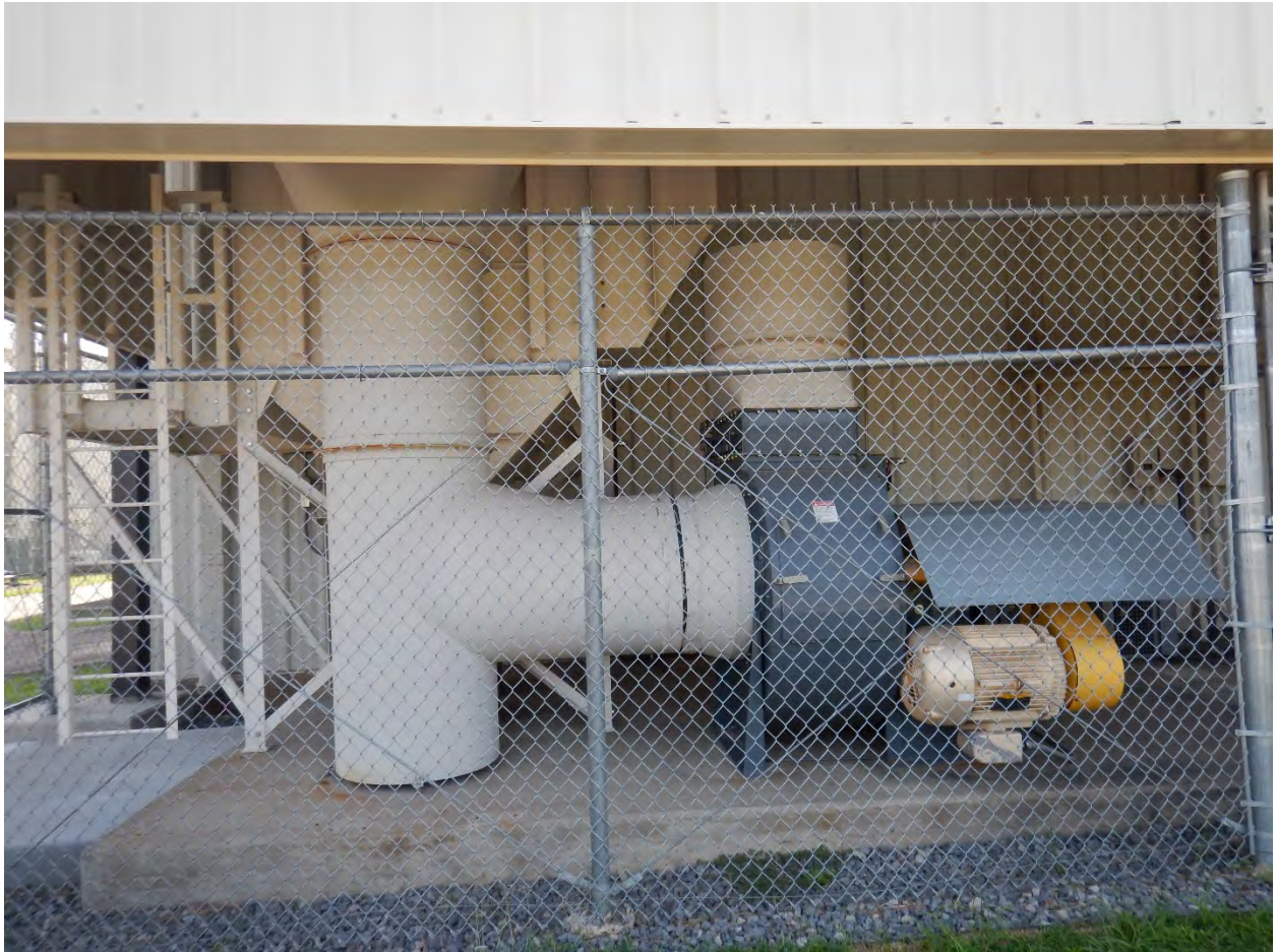
462 - Outside collection of bead blast at building 282
