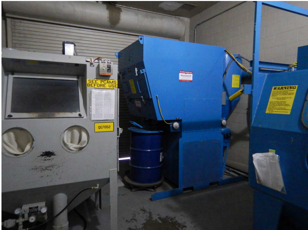
464 – Building 282 abrasive blast units
