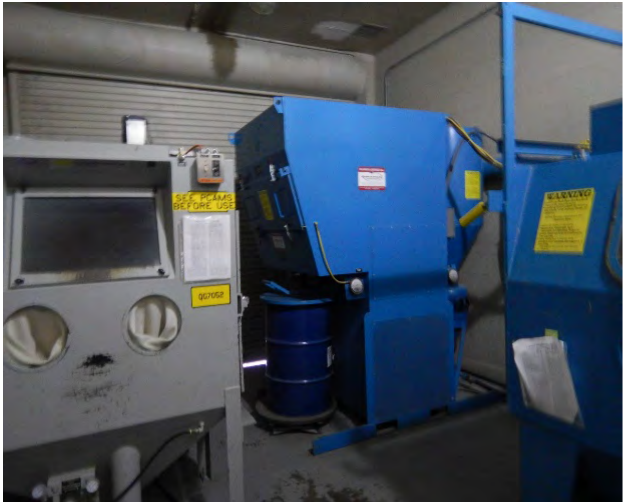
465 – Building 282 blast units
