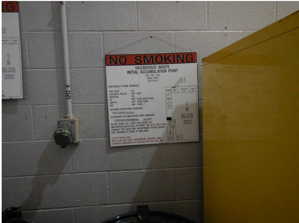
453 – Waste stream sign LRK-PRF-030 sign for SAA inside of building 282
