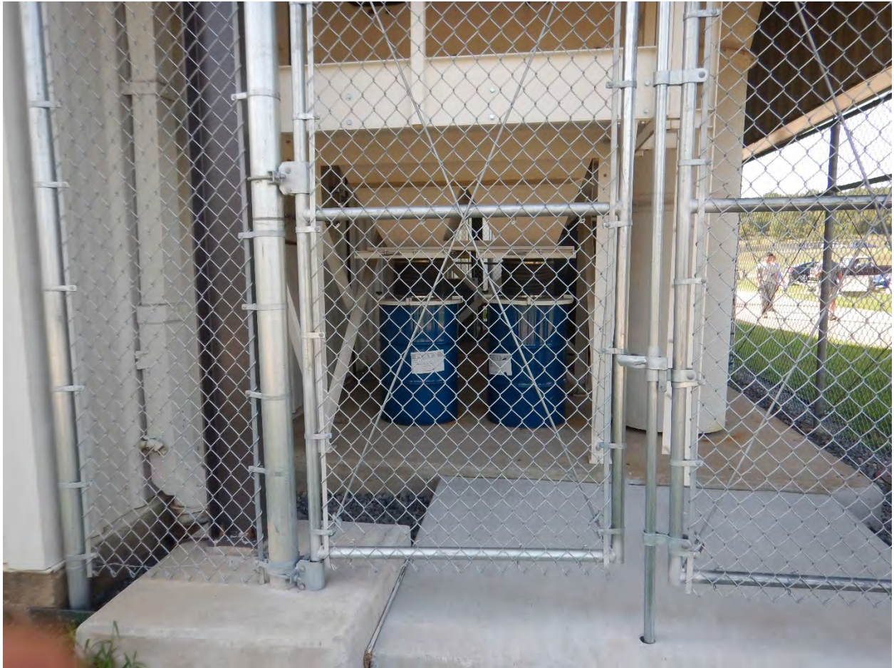
461 – Outside collection of bead blast at building 282
