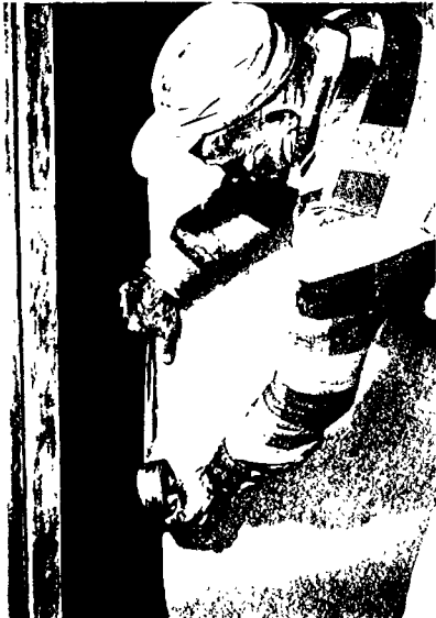
Tape all raw edges. No additional primer or sealer is necessary.
