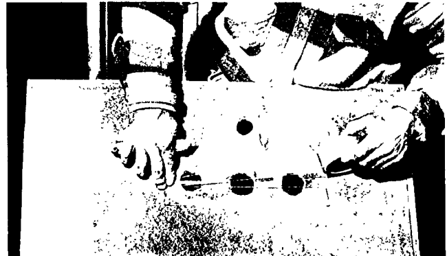
Apply strips of tape to back of Tile Backer Board across plumbing cut-outs.
