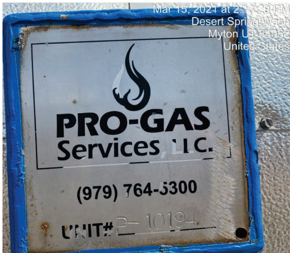
Photograph 10 – JT skid related
