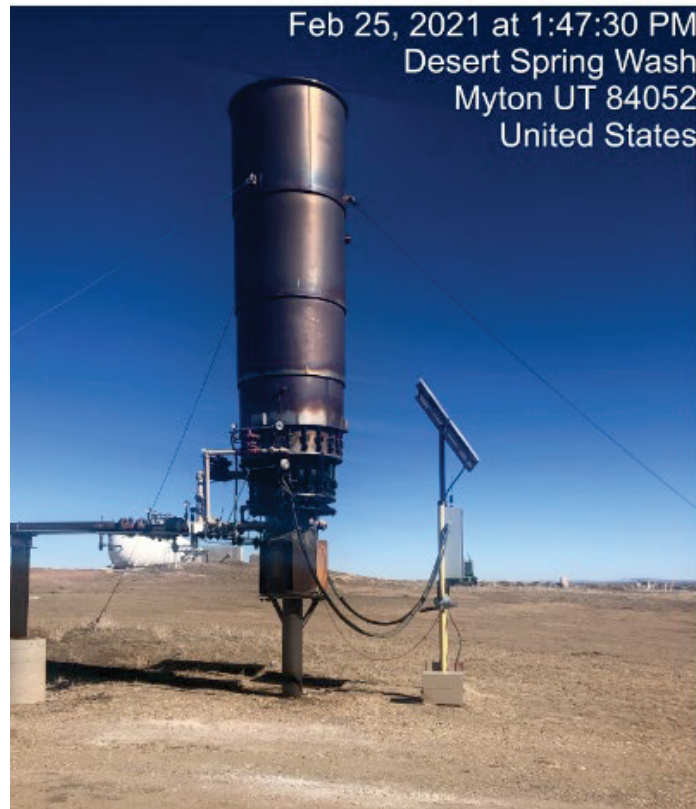
Photograph 13 – Thermal Oxidizer
