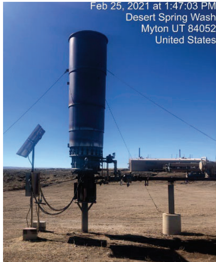
Photograph 12 – Thermal Oxidizer
