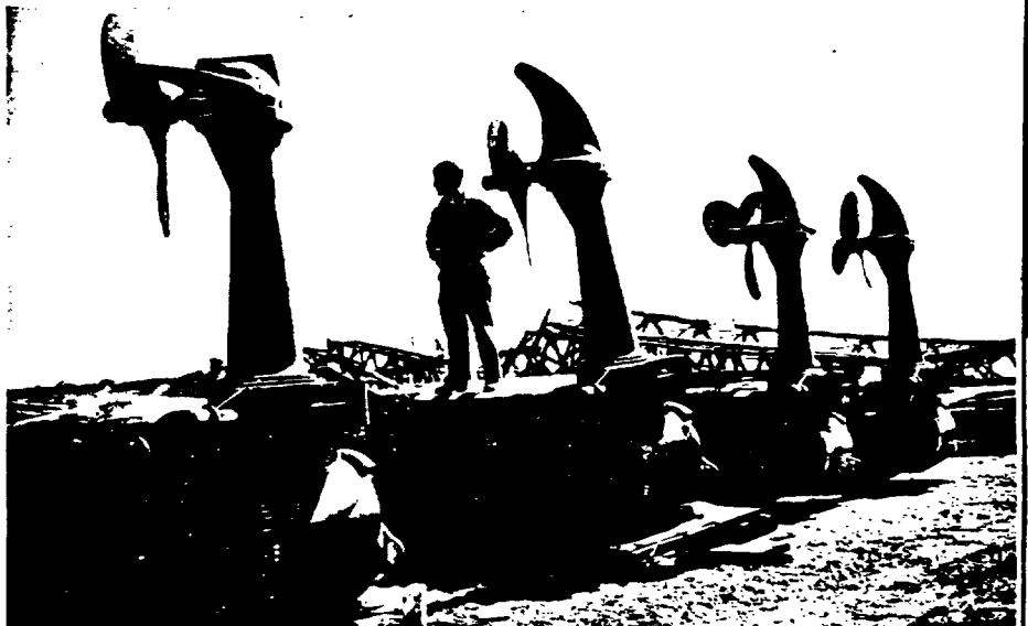
These giant outboard motors, in reality detachable power units, were used to help build rail spans across rivers
