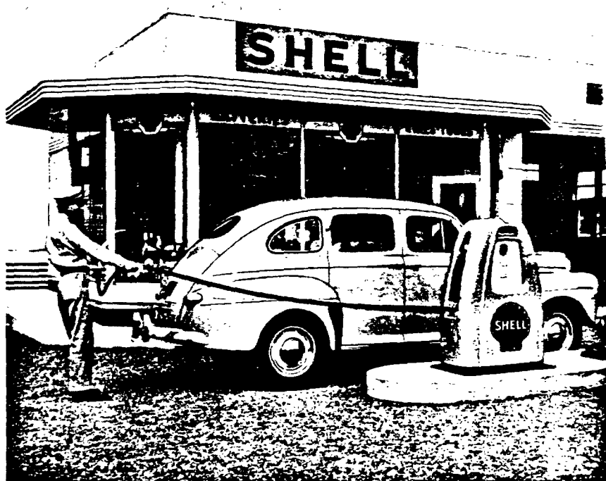
The new Shell station is of a strictly functional design. The pump is 54 inches high, with a hose 18 feet long
