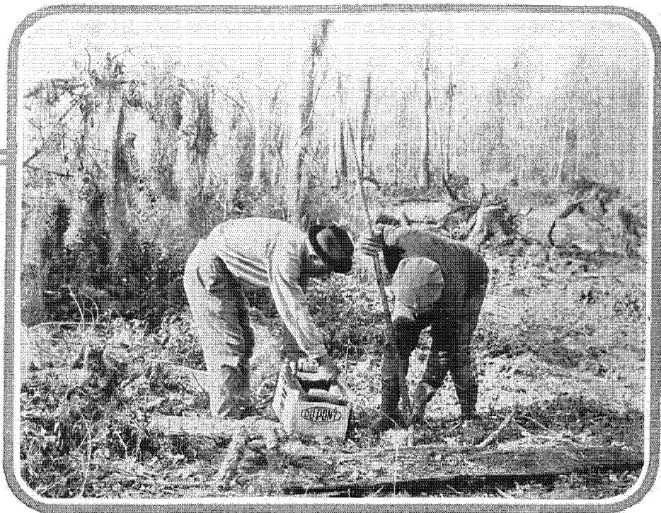
Loading du Pont dynamite along the right of way. The blaster is using a tamping stick, marked to insure uniform hole depth
