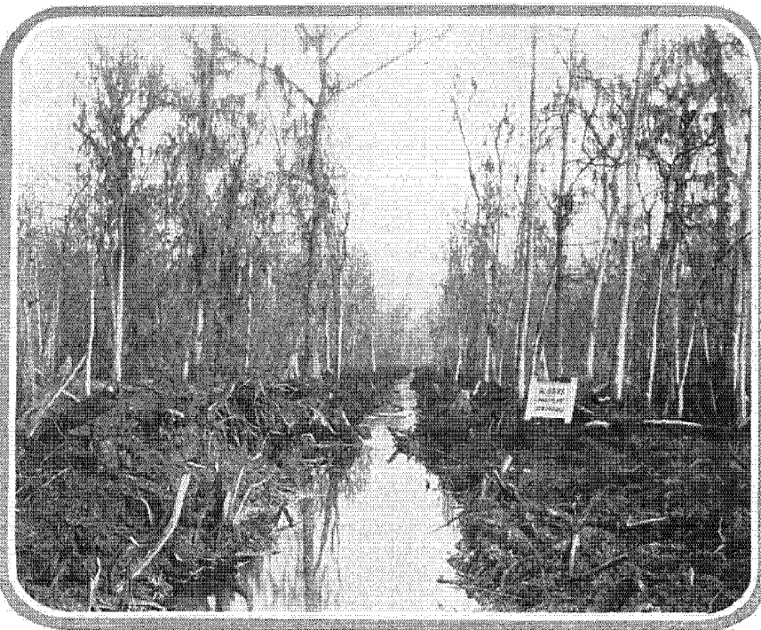
Water flowed through the new ditch a few moments after the blast. Note the absence of stumps and debris in the channel
