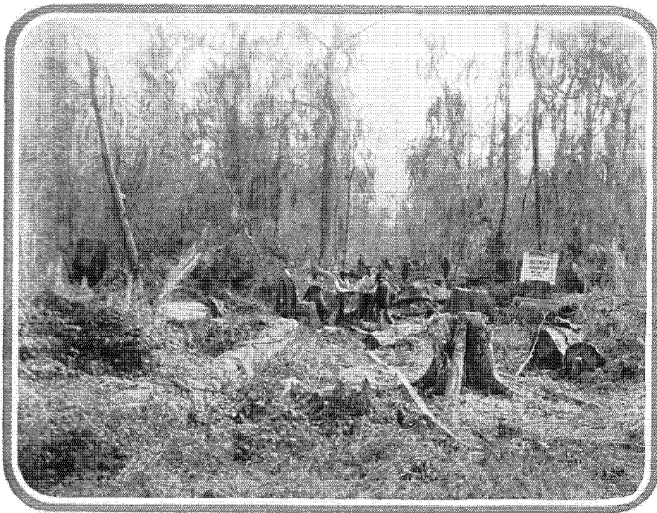
The ditch line after all trees had been cut down and the brush taken away. Logs and stumps shown here were lifted clear by the blast
