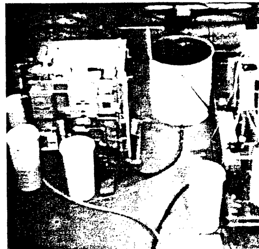
Water treatment pilot plant — Duluth, Minnesota (20 gal/min)
