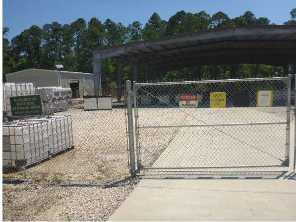
Photo 7: Chain link fence and signage securing entry to and identifying the hazardous waste Central Accumulation Area.
