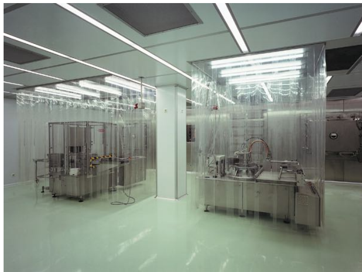
Figure 4.2: Highly clean cleanroom area separated with curtains.
