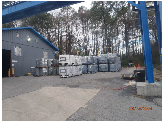
Picture 9 – Copper Plant Rework Area
