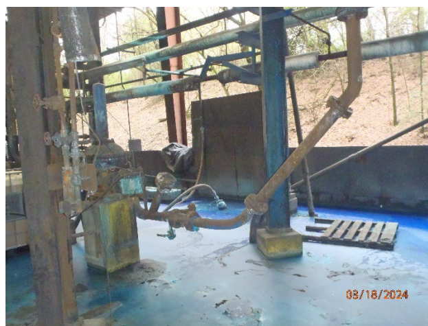
Picture 17 – Copper Oxide Plant sump area
