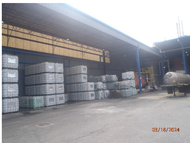
Picture 30 – Mix Plant Rework Area
