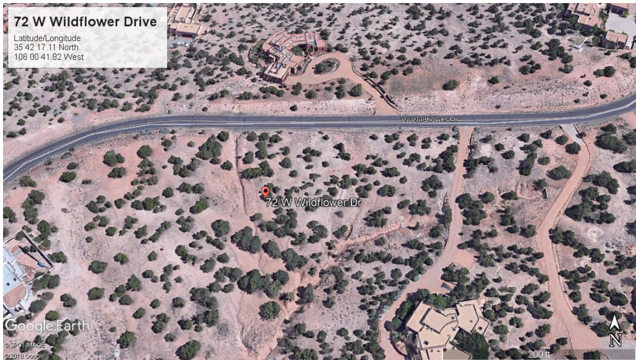
Aerial Image #1: Overall view of the 72 W Wildflower, Las Campanas Subdivision, Santa Fe, New Mexico. Aerial from Google Earth Maps.
