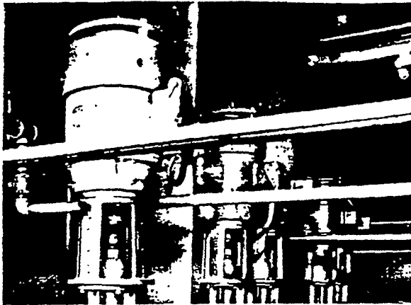
Advanced brass cleaning and pickling process at a leading metals producer and fabricator incorporates Deming pumps to create pressure for spraying the strip with the cleaning and pickling solutions.
