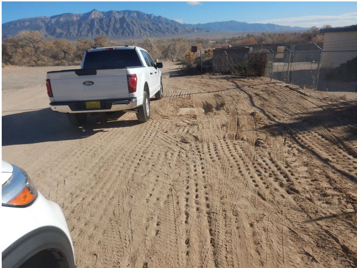
View looking approximately East adjacent to wire fabric perimeter fence of former WWTP #3 of the compacted land surface area where collapsed force was repaired. (DSCN2743) (12/23/2024) 2:43 PM. Photographed by D. Esparza
