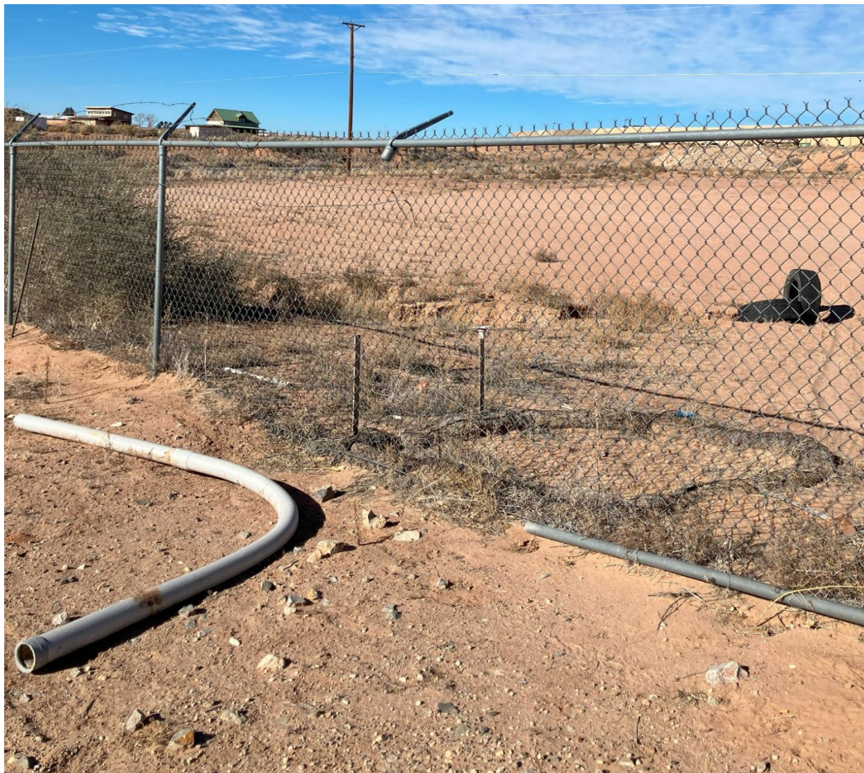
View looking north of LS-#15 damaged wire fabric perimeter fencing. NOTE: stormwater wattles outside fencing. (IMG_0537-cropped) Photographed by N. Fuad
