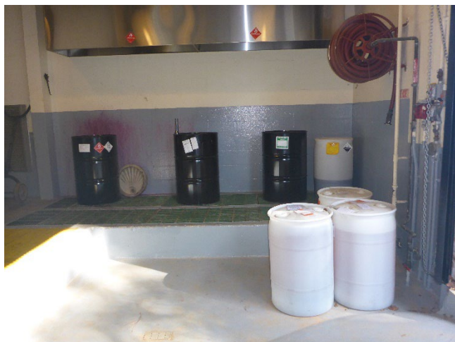
Photo 4: Two 55-gallon drums of waste flammable liquid (xylene, toluene); one 55-gallon drum labeled nonregulated waste; and one 30-gallon drum labeled hazardous waste flammable liquid (formaldehyde, methanol) in the flammable liquid bulking and barrel storage area in the TSD Building. One 30-gallon drum labeled toxic and corrosive hazardous waste containing ferrous ammonium sulfate, sulfuric acid, phosphoric acid, potassium permanganate and water; and two 30-gallon drums labeled toxic, flammable, and corrosive hazardous waste on the floor in the flammable liquid barrel storage and bulking area.
