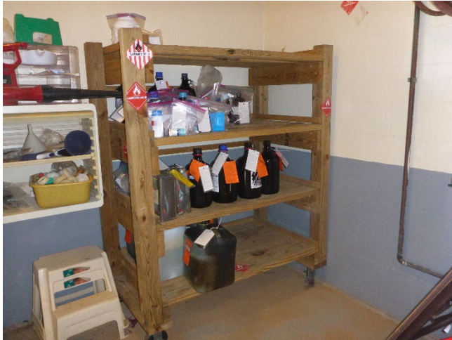
Photo 1: Waste containers on the wooden shelves at the incoming waste processing area in the TSD Building.
