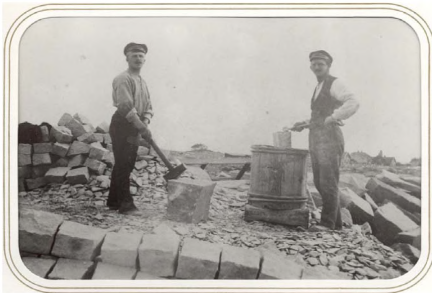
Figure 3. Granite cutters (about 1925). The subsequent introduction of power tools and enclosures to reduce the effects of bad weather, led to large increase in the number of cases of silicosis and silico-tuberculosis among granite cutters. Today the trade is virtually extinct.
