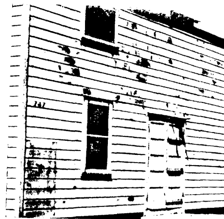
FIGURE 10.—Typical discoloration of paint. Before repainting, surface should be scrubbed with alkaline cleaner, for example, trisodium
