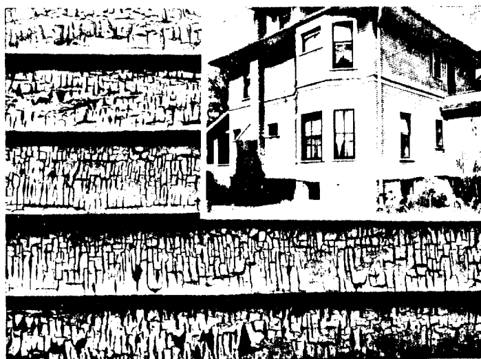
FIGURE 27.— Example of alligatoring.
