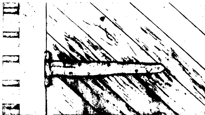
FIGURE 14.—Illustration of how painted wood starts to decay around a hinge, which holds water.
