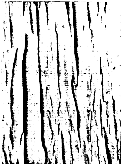
FIGURE 19.—Details of paint cracking on exterior of wood building.
