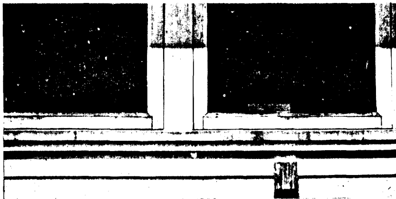
FIGURE 12.—Discoloration of light-colored paint underneath fly screens, due to the corrosion of the screens.
