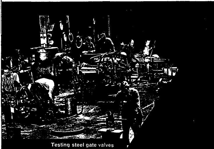
Testing steel gate valves
