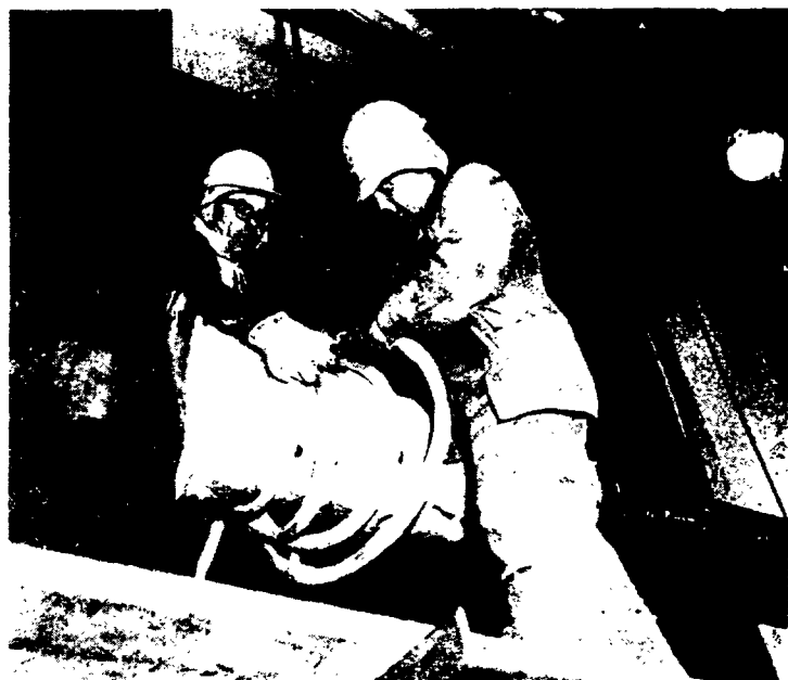
Figure 3. Workmen coiling induction cable around crossover pipe insulated with jacketed Kaowool blanket. The asbestos sleeve insulation on the cable is protected from excessive heat by the blanket.
