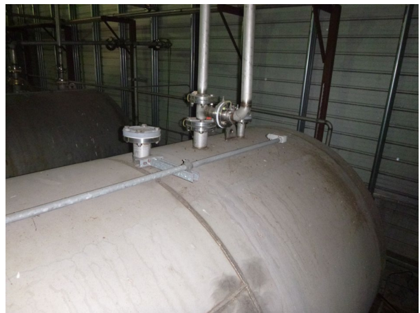
Photograph 30: Hazardous Waste CAA Tank TK503.
