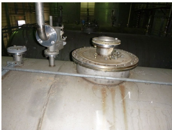
Photograph 29: Hazardous Waste CAA Tank TK503.
