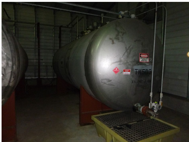
Photograph 33: Hazardous Waste CAA Tank TK503.
