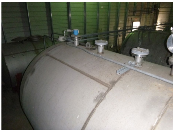
Photograph 28: Hazardous Waste CAA Tank TK503.
