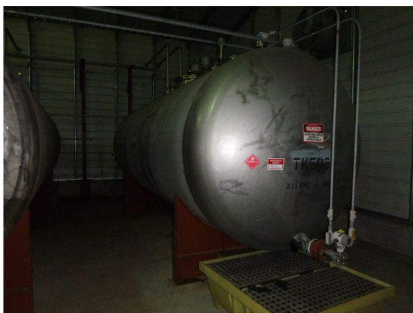
Photograph 34: Hazardous Waste CAA Tank TK503.
