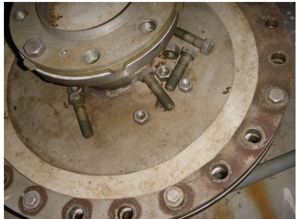
Photograph 31: Hazardous Waste CAA Tank TK503.
