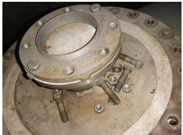
Photograph 32: Hazardous Waste CAA Tank TK503.
