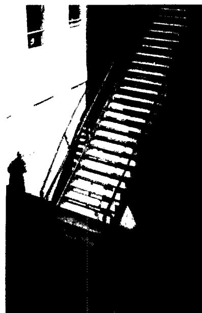
Resurfacing worn metal and concrete fire escape steps at a public school in St. Paul, Minn., with an emulsified asphalt mortar has reduced a hazard.
