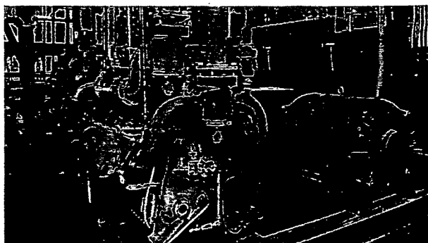
Two Frick NEW "ECLIPSE" Compressors, each with 9 Cylinders, Air Condition Weingarten's Supermarket at Houston.
