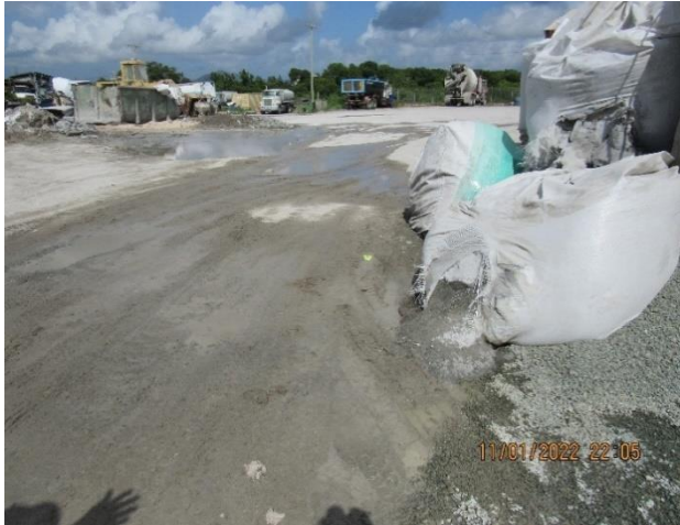
IMG 765 -Close-up of cement and gravel in the path of stormwater flow that drains toward the retention
