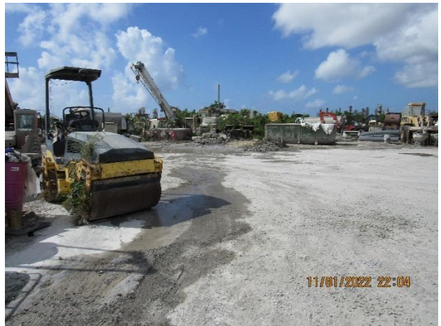
IMG 764 -Path of dry-weather flow from the ready-mix concrete plant running across the yard towards the retention pond.
