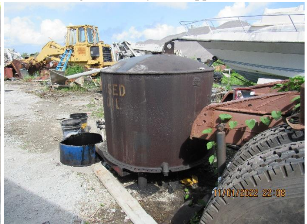
IMG 769 -Container in which the Facility's used oil is collected and stored on-site. Improper housekeeping conditions observed and documented.
