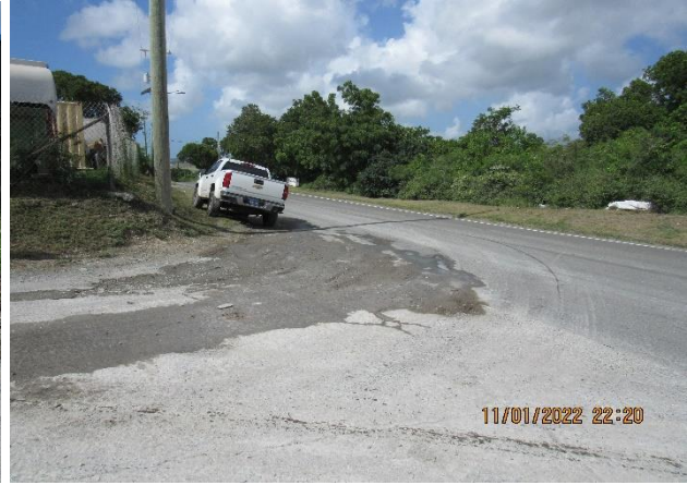
IMG 777 -Dry-weather flow leaving the Facility and out into the public road.
