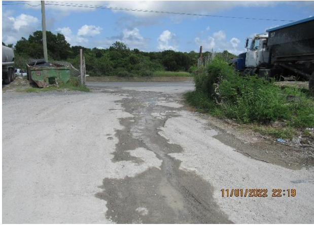
IMG 775 -Dry-weather flow being discharged from Facility through the lower entrance/exit.
