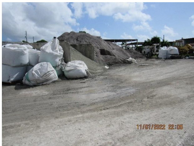
IMG 767 -Bags of cement stored immediately next to aggregate (sand & gravel) cells. Some bags were ripped, with cement spilled onto ground.
