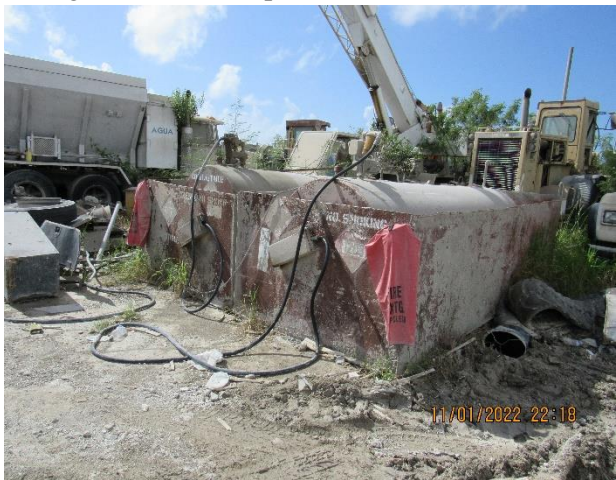
IMG 772 -Facility's fueling terminal situated in path of stormwater flow. No containment in area where vehicles are staged for fueling service.
