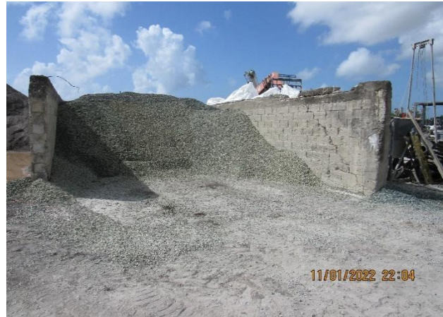
IMG 762 -Storage cell with gravel situated next to sand storage. Storage area exposed to stormwater runoff flow, leading to wash-off of material.
