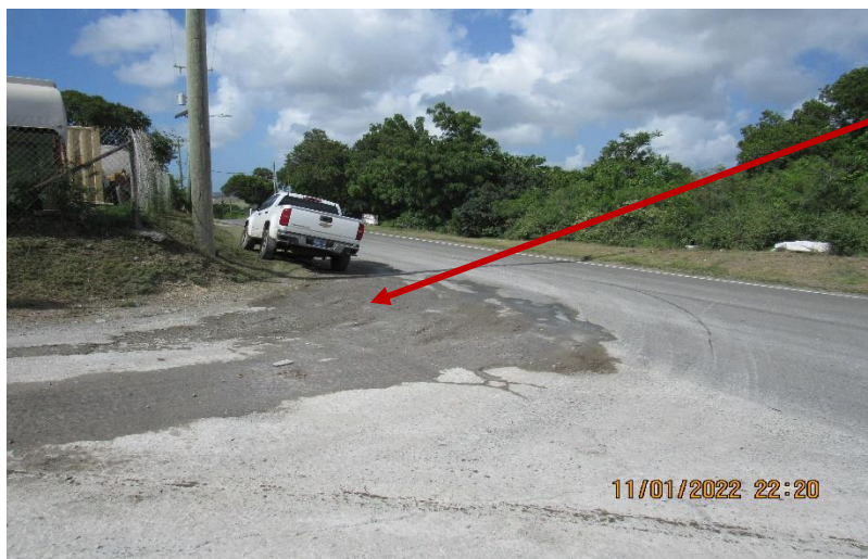
IMG 777 - Discharge point where stormwater runoff flow from the central area (shallow retention pond) combined with flow from the northwestern (truck parking area) of the Facility and discharged into the public road through the lower entrance/exit. Stormwater flow drains into Fig Tree Ghut, and Cane Garden Bay downstream.
