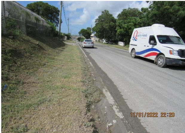
IMG 778 -View of dry-weather flow event occurring and running along left side of the road downhill in the stormwater flow path along the road.
