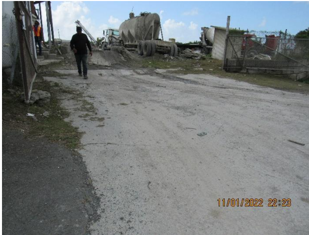
IMG 781 -View of the ready-mix loading bay, upper entrance/exit and stormwater flow path out of the Facility and into the public road.
