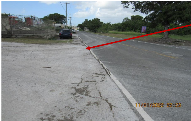
IMG 782 -Discharge point where stormwater runoff flow from around the Ready-Mixed Concrete Plant loading bay and vicinity of the Administrative Building are combined and discharged into the public road through the upper entrance/exit. Stormwater flow drains into Fig Tree Ghut, and Cane Garden Bay downstream.
