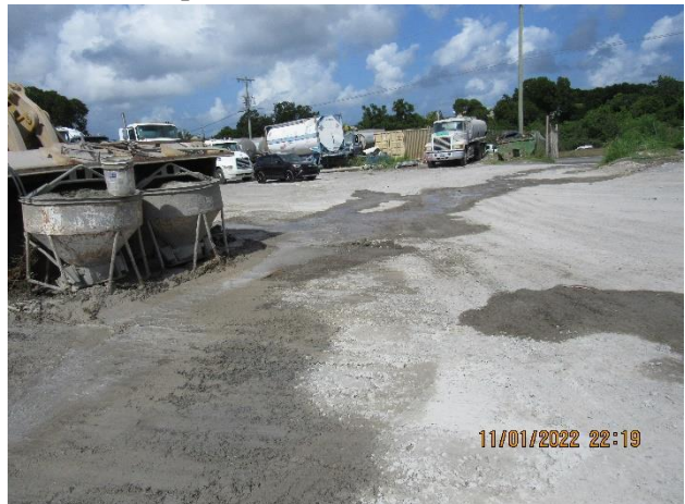
IMG 774 -Dry-weather flow the pond drains away from the pond across the yard towards the lower entrance/exit, transporting pollutants (e.g., industrial wastewater).
