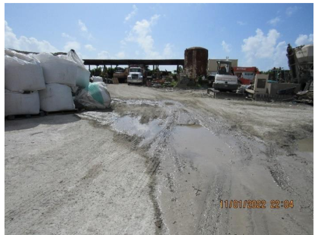
IMG 768 -Observed that the cement bags and spilled cement sits in the stormwater flow path. Cement spilled will be washed-off by stormwater runoff.
