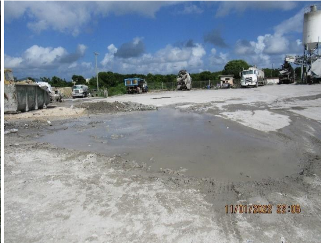
IMG 766 -Close-up retention pond, and deposited spent concrete used to form a berm.
