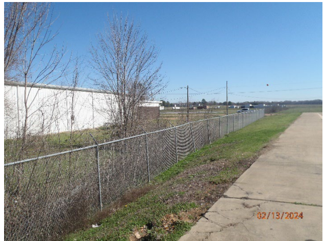
Picture 17 – Tank Secondary Containment near unnamed tributary to Town Creek
