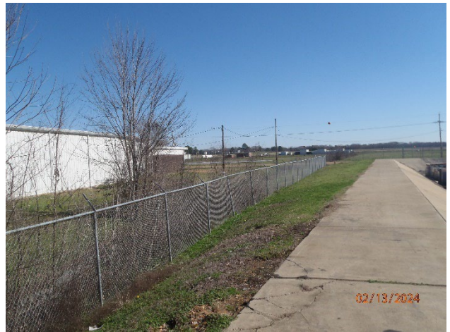
Picture 18 – Tank secondary containment near unnamed tributary to Town Creek
