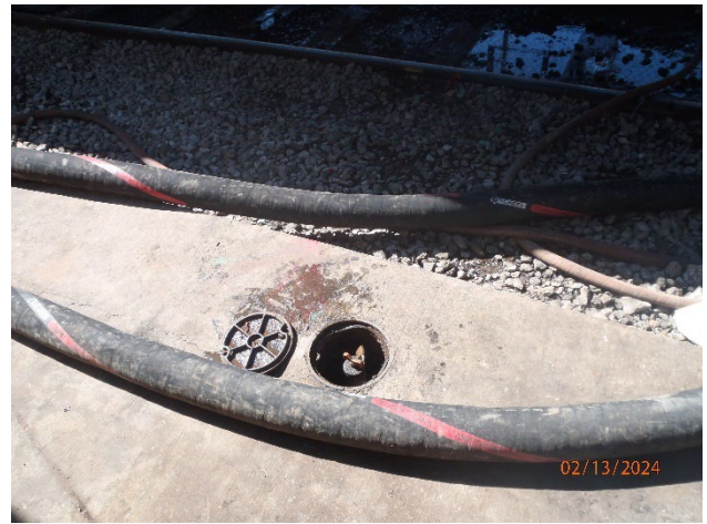
Picture 4 – Monitoring Well 7 in AOC C
