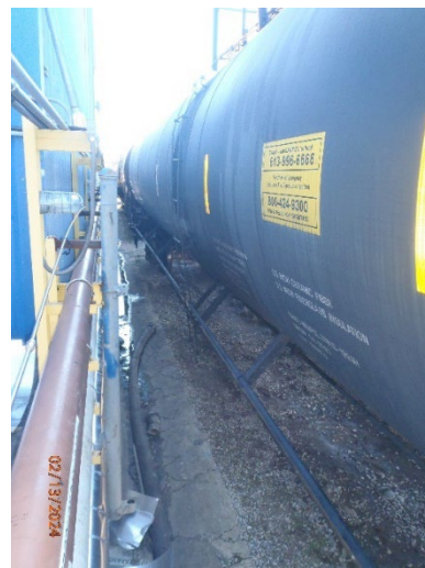
Picture 11 – Internal Railway – area of 2020 Diesel Release
