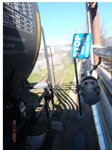
Picture 12 – Internal Railway – area of 2020 Diesel Release
