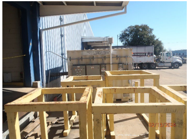
Picture 23 – Vapor Intrusion Building and Alarms
