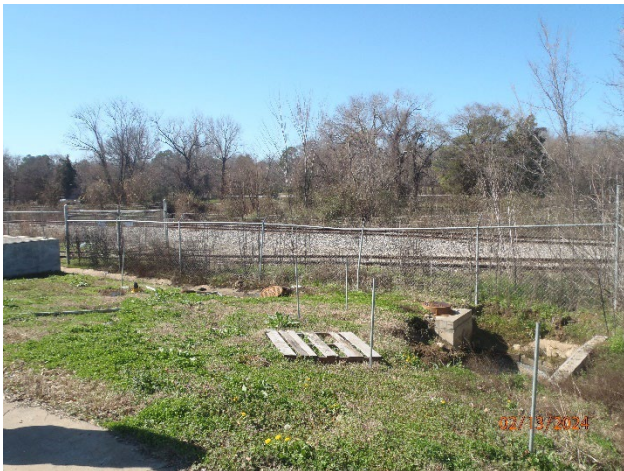
Picture 20 – Railway discharge to Oil Water Separator and Sump Collection Basin
