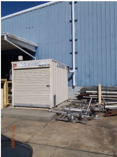
Picture 25 – Vapor Intrusion Building
