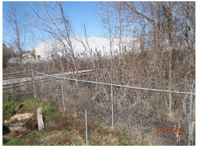
Picture 16 – Sump Collection Basin near unnamed tributary to Town Creek
