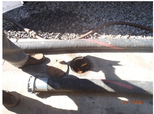
Picture 5 – Monitoring Well 16 in AOC C
