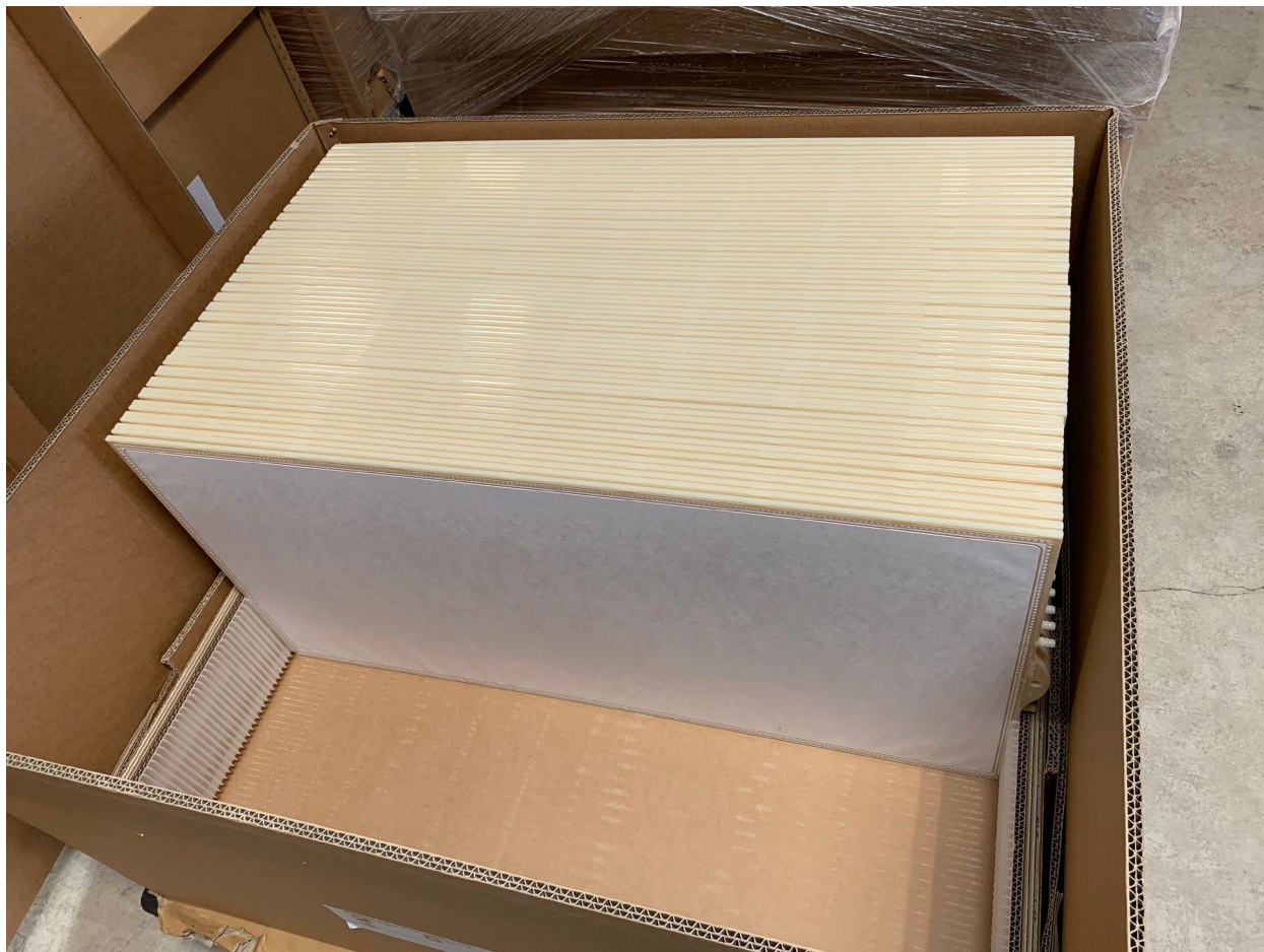
Replacement membrane cartridges awaiting installation. (IMG0143). September 13, 2022. Photographed by D. Esparza
