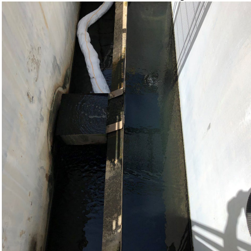
Photo #2. Samples were collected from Outfall 002 monitoring location.
