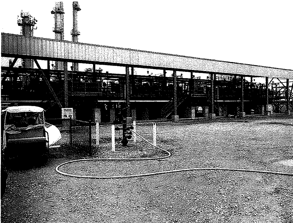
Flare Gas Recovery-Compressors
