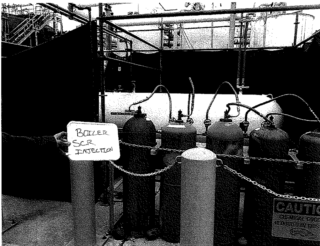
Boiler SCR Injection
