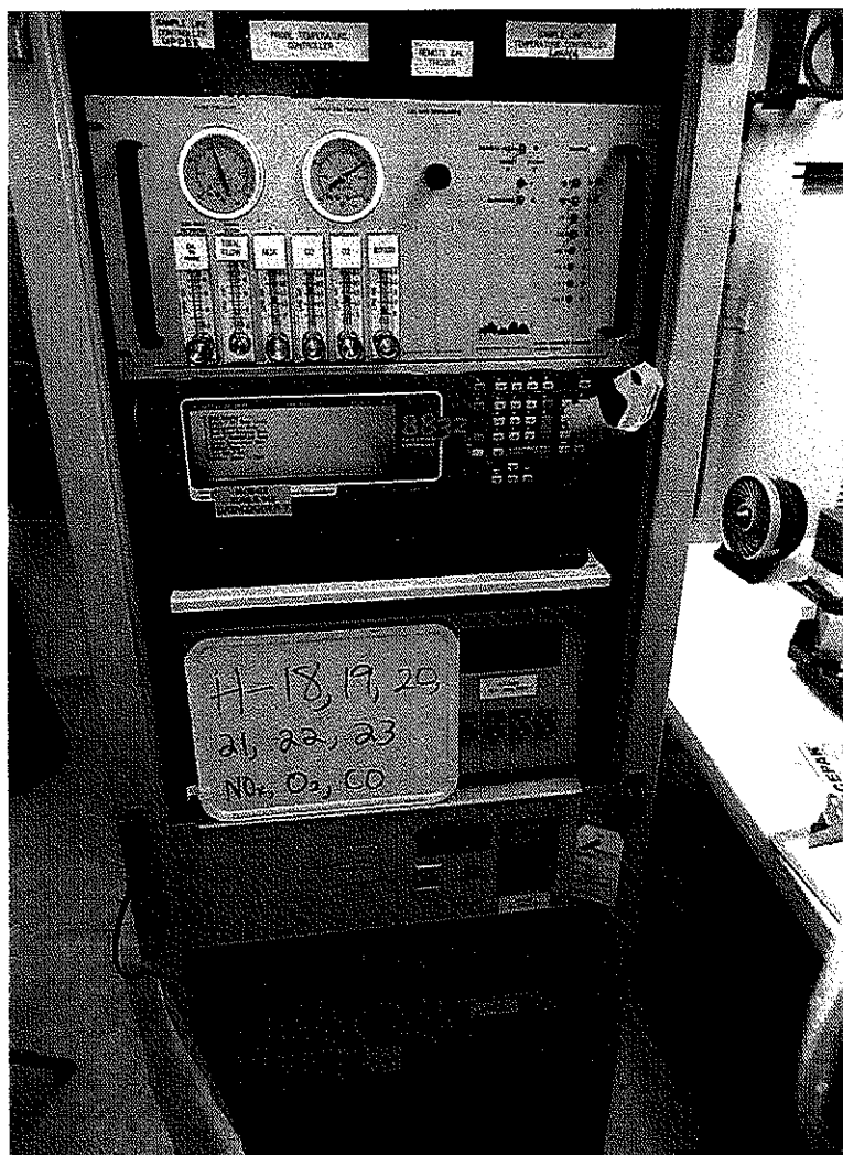
H-18, 19, 20, 21, 22, 23 (Combined Stack) NOx, O 2 , CO CEMS
