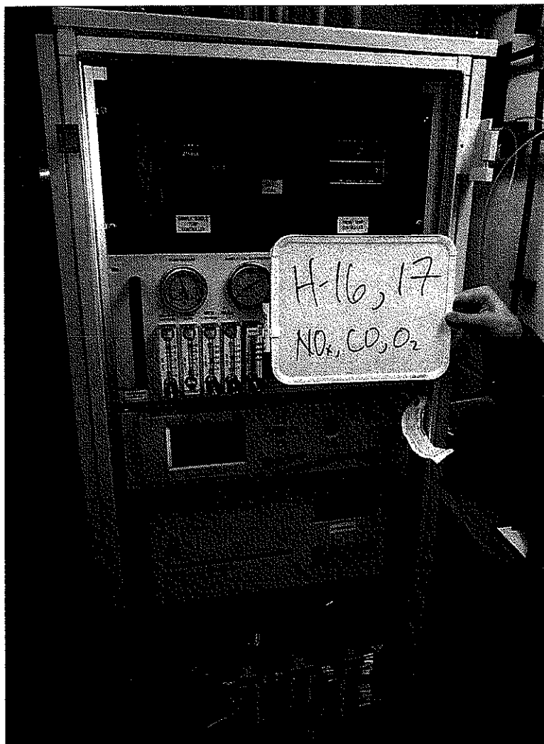
H-16/H-17 (Combined Stack) NO x , CO, O 2 CEMS
