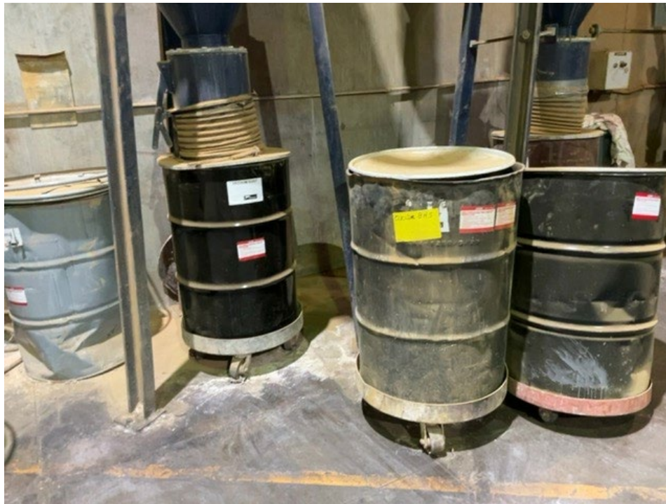
Photo 21 – Drum accumulating nonRCRA hazardous baghouse dust in the Oxide Area.
