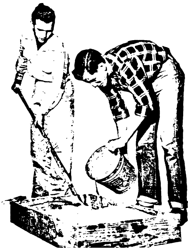
FIRST STEP in the manufacture of the C-EZ Company's lawn markers was mixing the concrete
