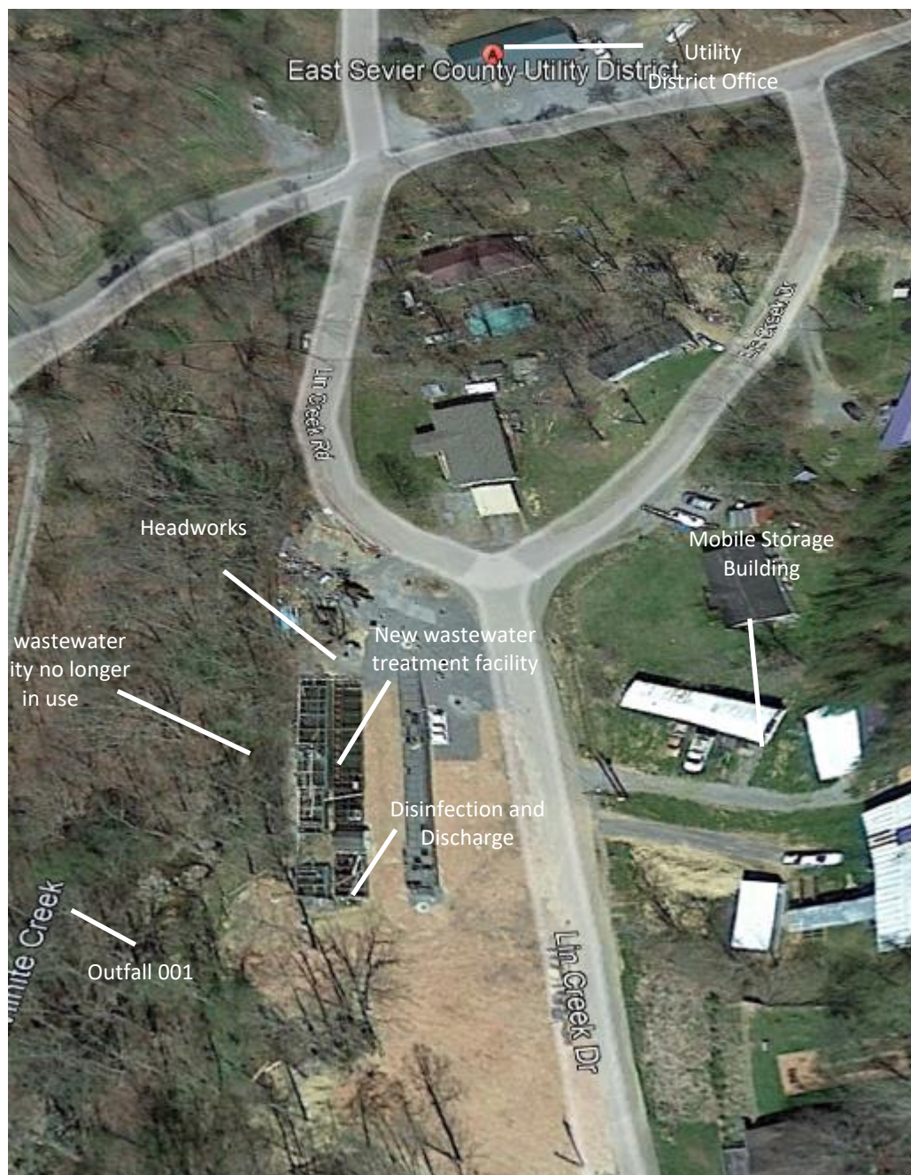
Figure 1: Aerial View of the ESCUD STP dated April 2022.
