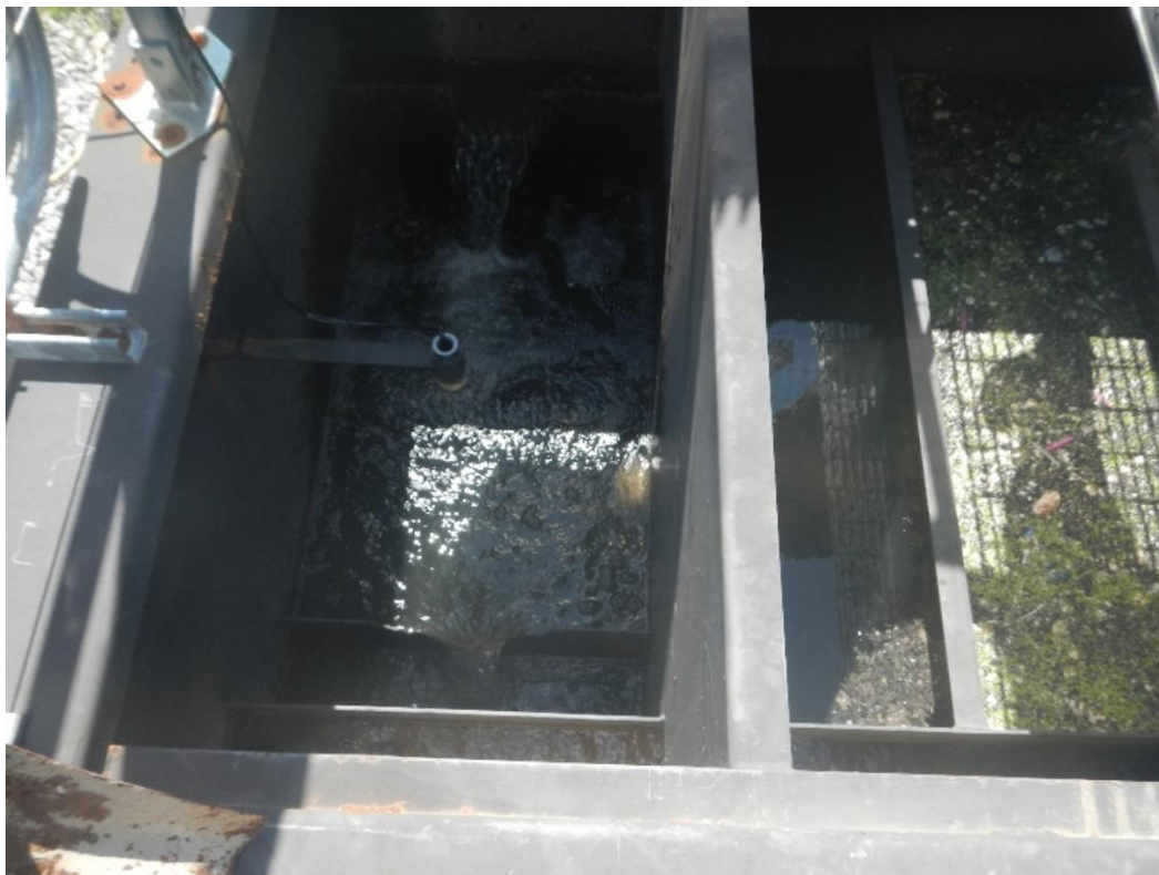
Photo 5: Turbulent flow under ultrasonic flow meter
