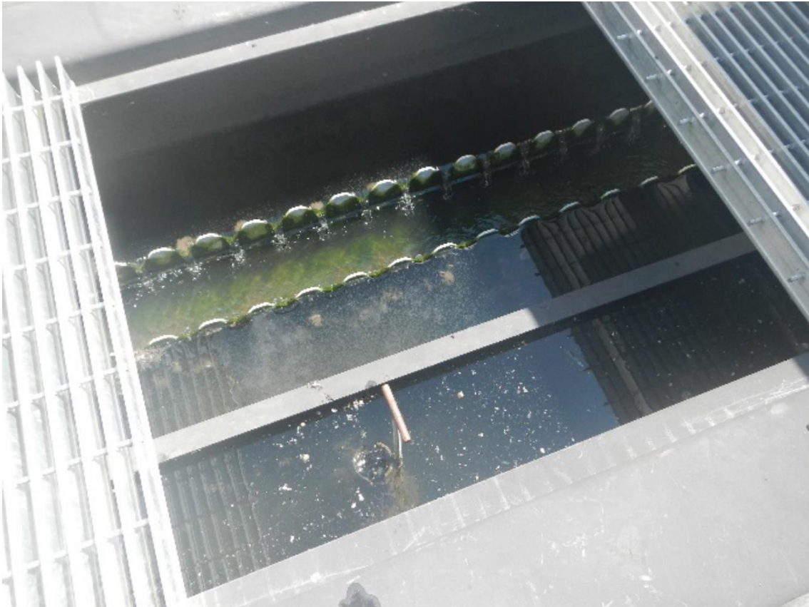
Photo 3: Algae and vegetation on weirs within clarifier.
