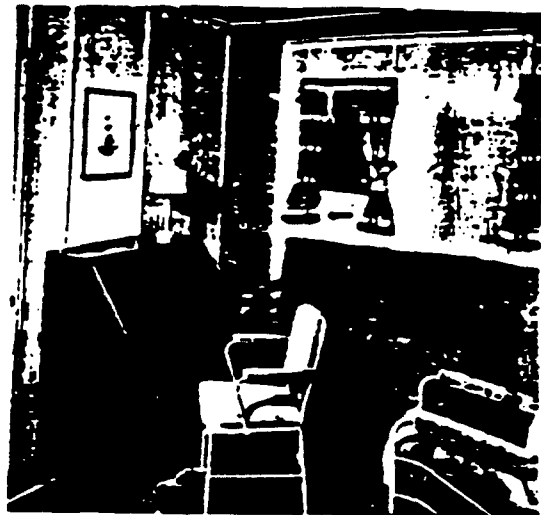
Cabin finish of wood-veneered Marinite bulkheads with painted J-M Marine Sheathing ceiling
