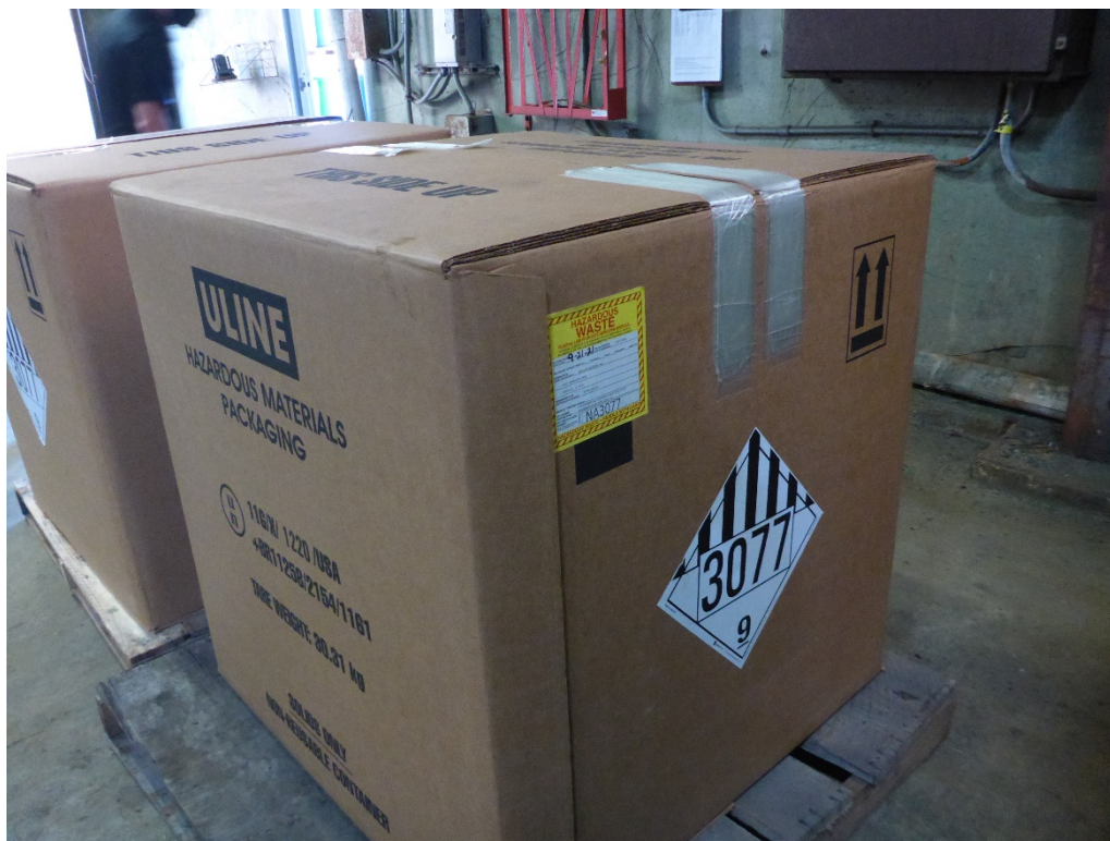
Photo 4: Two cubic yard boxes of used gloves, respirator cartridges and other PPE, empty product bags and contaminated trash in the CAA. Each box was labeled D007 / D008 hazardous waste solid and identified with a DOT class 9 hazard placard. One box was dated 11/16/2021 and the other was dated 09/21/2021.
