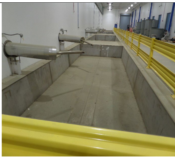
Corning. Salt Shed. The inspectors observed four stainless-steel lined concrete pits (pit) that store potassium nitrate (D001) generated from the ion-exchange unit IOX-104. Photograph 4 taken at 11:55 a.m.
