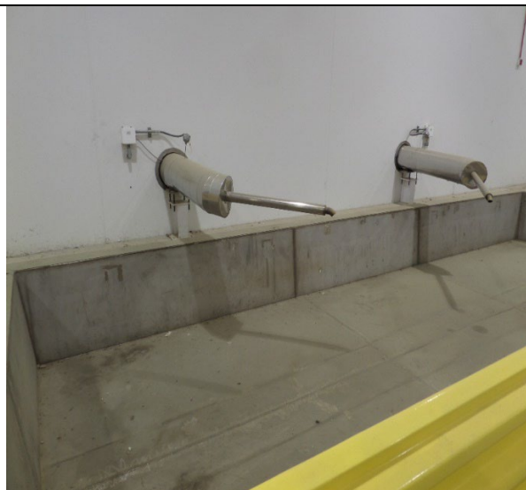
Corning. Salt Shed. The inspectors observed four stainless-steel lined concrete pits (pit) that store potassium nitrate (D001) generated from the ion-exchange unit IOX-104. Photograph 2 taken at 11:55 a.m.
