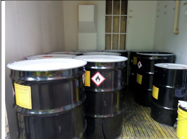
Corning. Outdoor CAA. The inspectors observed the container aisle space was not maintained. Photograph 9 taken at 12:22 p.m.
