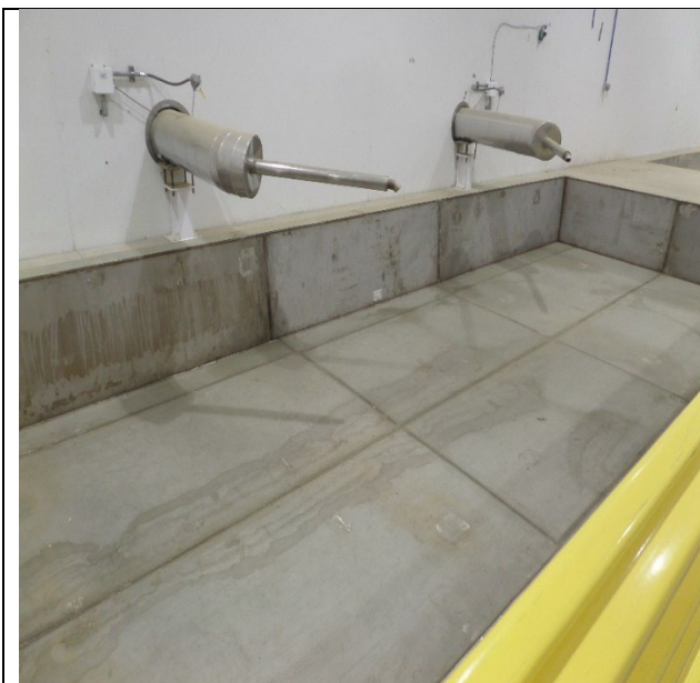
Corning. Salt Shed. The inspectors observed four stainless-steel lined concrete pits (pit) that store potassium nitrate (D001) generated from the ion-exchange unit IOX-102. Photograph 5 taken at 11:57 a.m.
