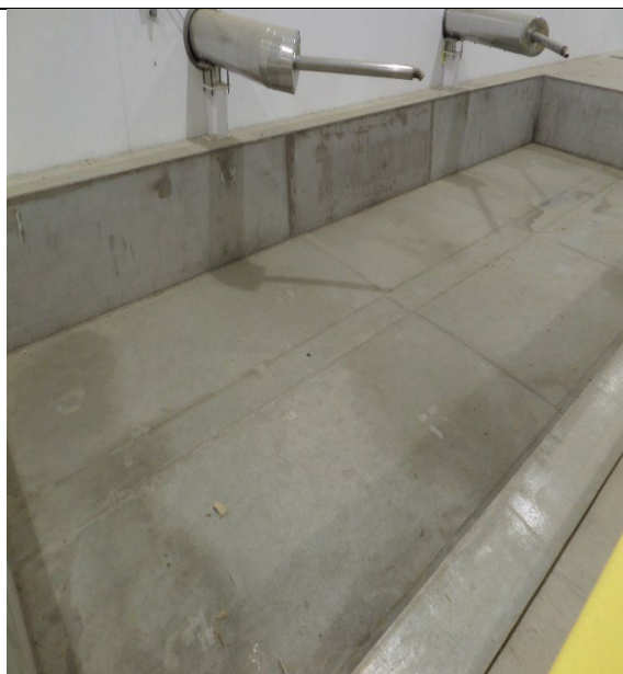
Corning. Salt Shed. The inspectors observed four stainless-steel lined concrete pits (pit) that store potassium nitrate (D001) generated from the ion-exchange unit IOX-103. Photograph 6 taken at 11:57 a.m.
