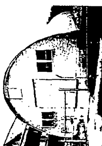
Sheet steel structures are given longer life and lower inside temperature with Asphalt Protective Coating followed by Flintkote Aluminum Paint.
