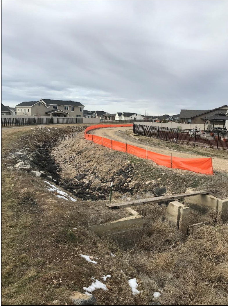
Photograph 1. View, facing west, of the Kuna Canal as seen from North Sailer Way. Note the silt fence located north of the Kuna Canal.
