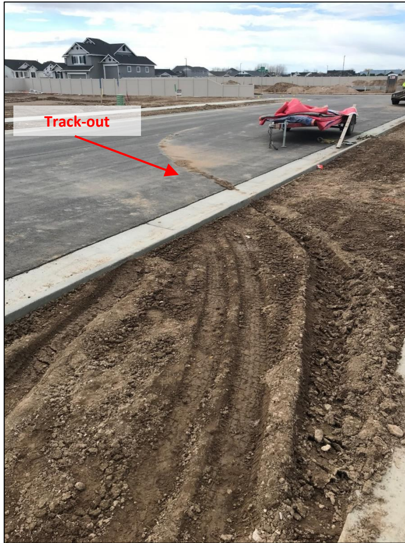
Photograph 3. View, facing southeast, of sediment track out onto North Hose Gulch Avenue due to access by vehicles or construction equipment at non-designated entrance/exits.
