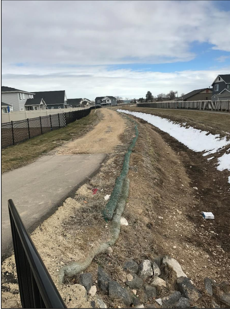
Photograph 2. View, facing east, of the Kuna Canal as seen from North Sailer Way. Note the fiber roll located north of the Kuna Canal.
