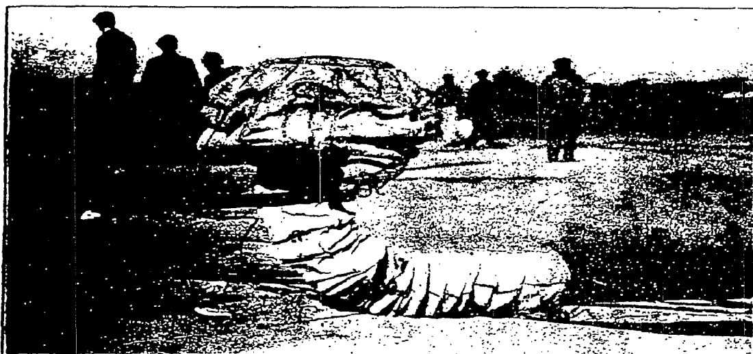
Asbestos tube contracted.
