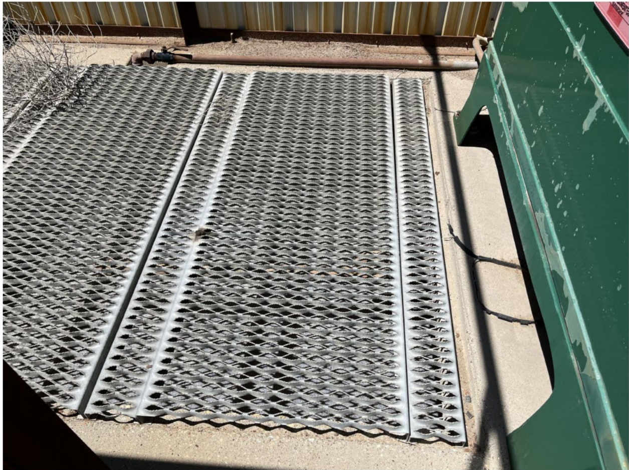
View of "diamond plate" steel grating covering the wastewater treatment headworks. (IMG_0081). Photographed by D. Esparza
