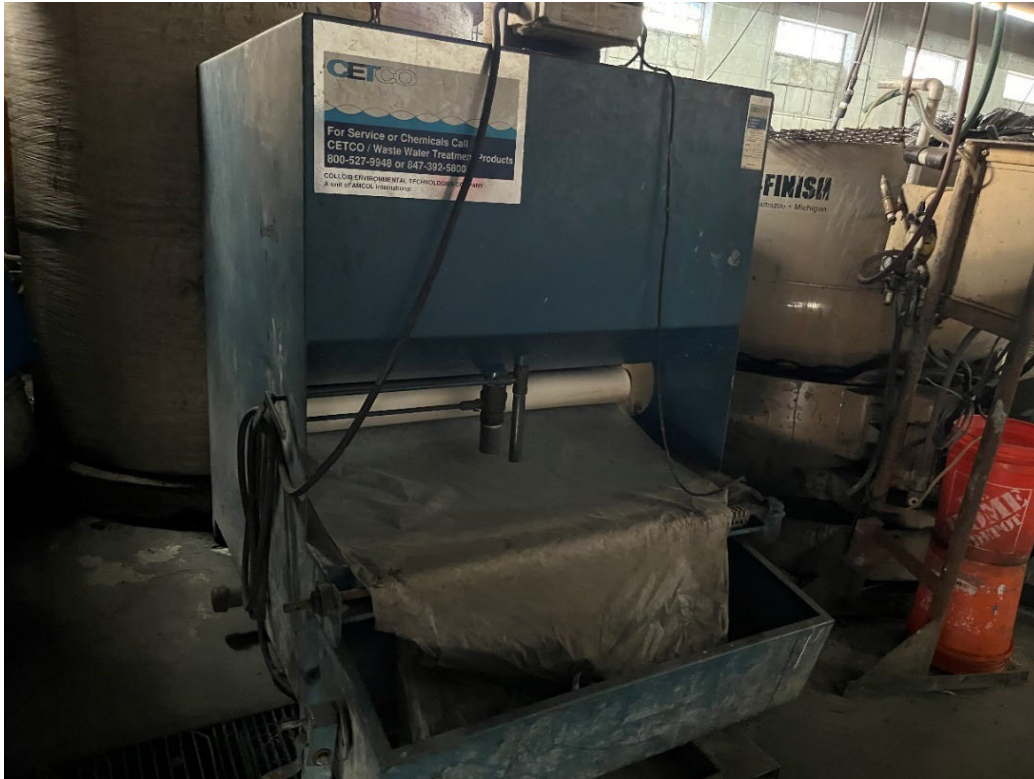
Photo #5. Wastewater is pumped into on-site portable treatment system.
