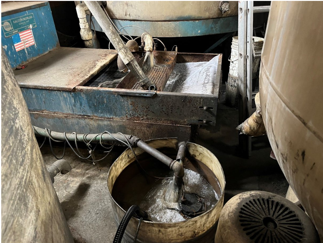
Photo #4. Solids are removed and the filtrate flows into the plastic junction container.
