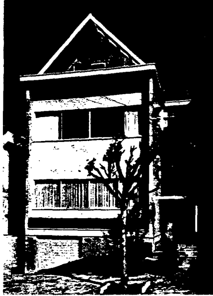
Simplicity of contour and surface and form distinguish the exterior of the completed remodeling job. Notice that part of the basement became a garage.
