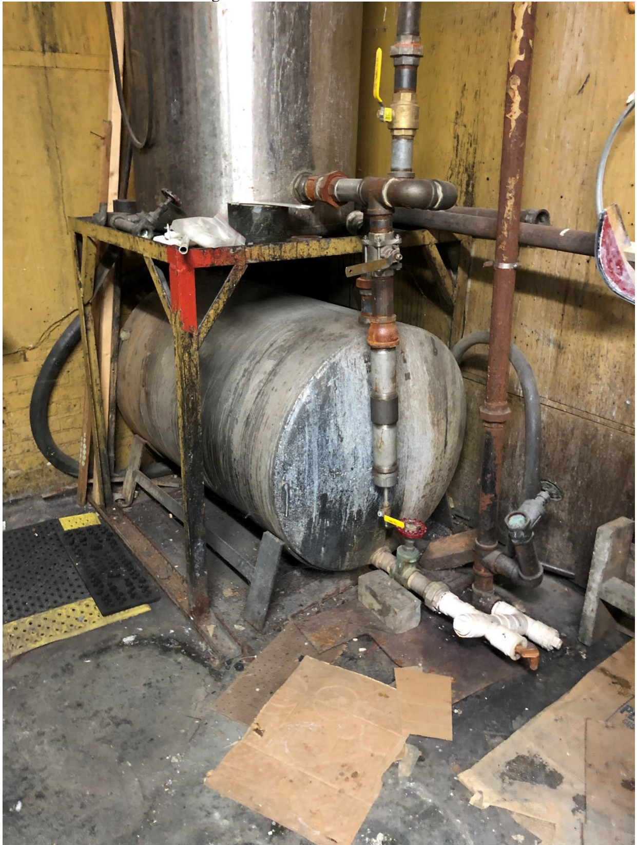
Photo #4: View of the receiving tank.
