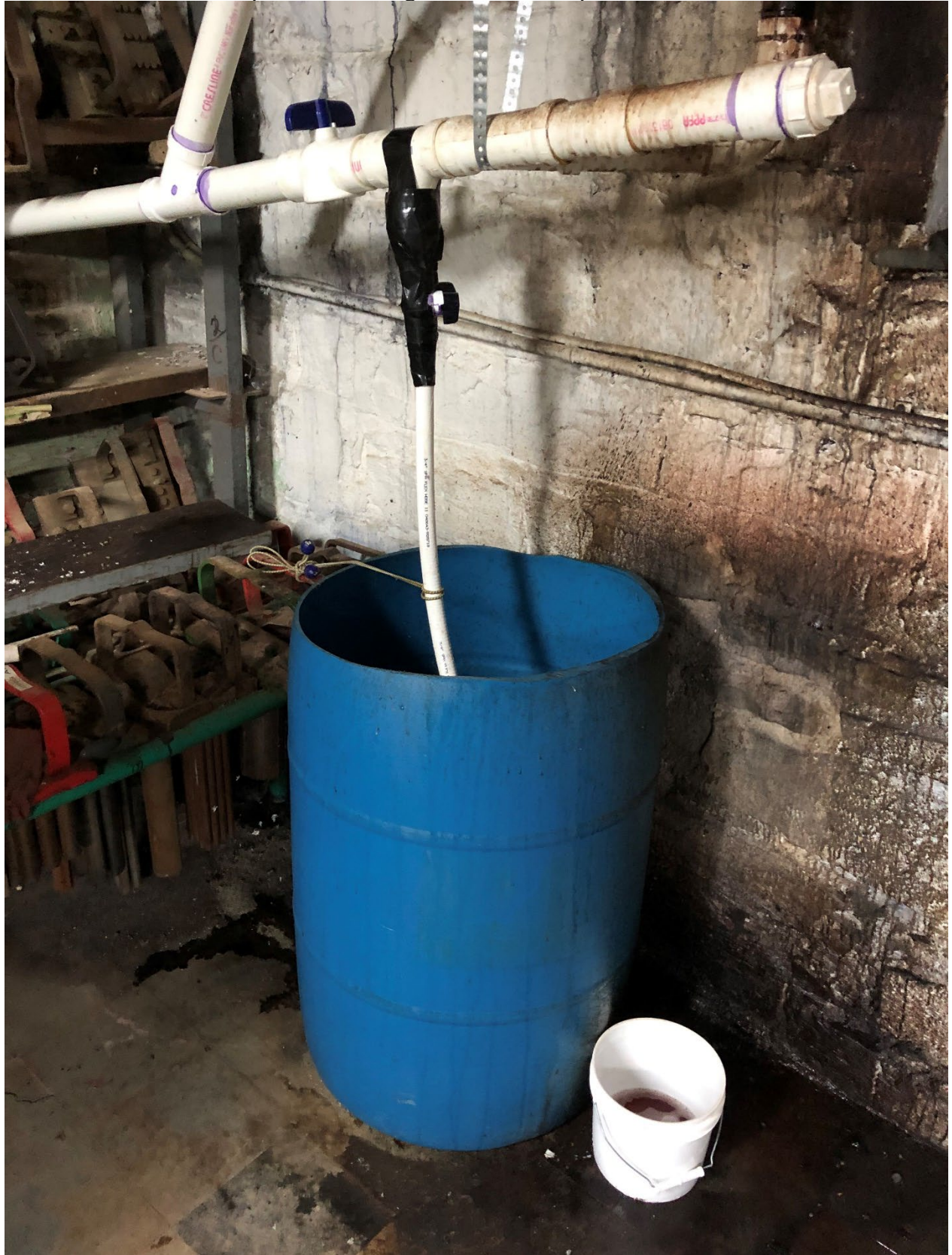
Photo #5: View of the tap on the discharge line where samples were collected.
