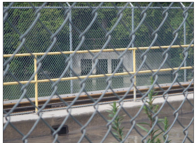
Photograph 80. DTE - Monroe Plant DSCN0166.JPG Description: View, facing west, of the wastewater treatment plant outfalls into the discharge canal.
