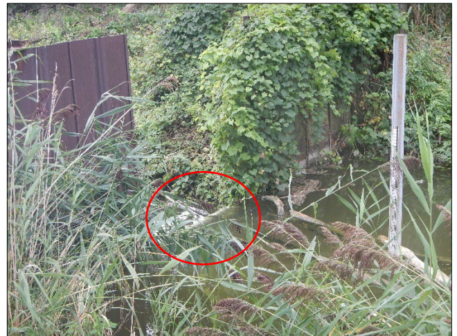
Photograph 64. DTE - Monroe Plant DSCN0150.JPG Description: Closer view facing southeast of the Outfall 001F staff gage and effluent sampling weir (circled).
