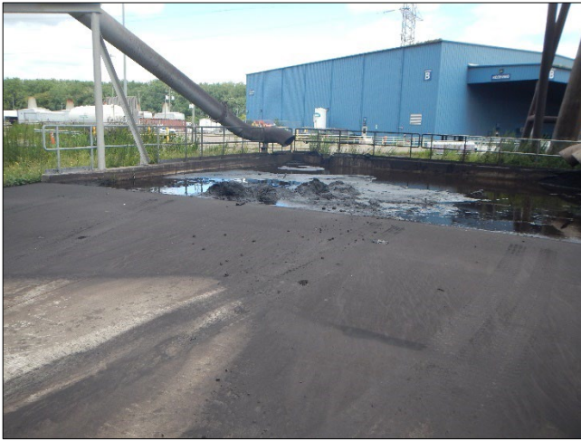
Photograph 89. DTE - Monroe Plant DSCN0175.JPG Description: View, facing north, of the Coal Fines Washdown Pond.
