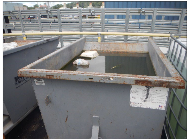
Photograph 96. DTE - Monroe Plant DSCN0182.JPG Description: Up-close view of hoppers seen in Photograph 92.
