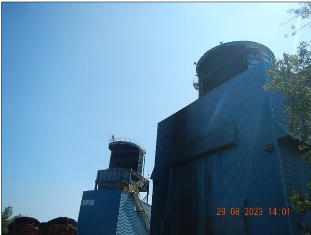
Photograph 6. DTE - Monroe Plant DSCN0092.JPG Description: View, facing southeast, of coal transfer houses.
