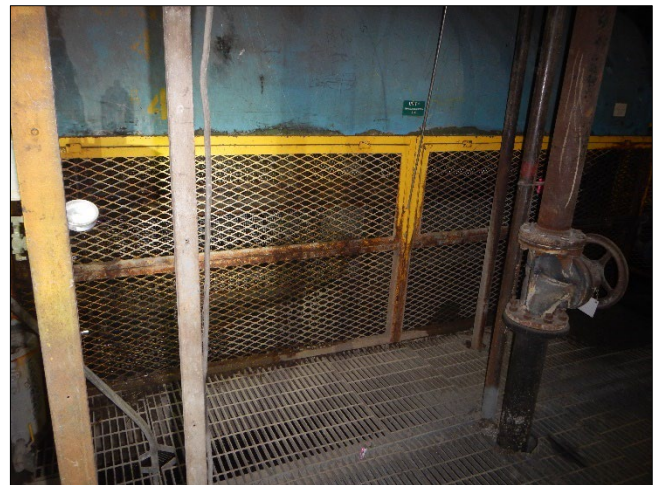
Photograph 88. DTE - Monroe Plant DSCN0174.JPG Description: General view inside the Number 3 and 4 screenhouse building.
