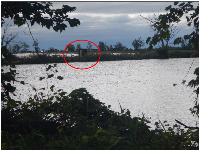
Photograph 70. DTE - Monroe Plant DSCN0156.JPG Description: View, facing east, across the Discharge Canal from Outfall 001F towards Outfall 001B (circled).
