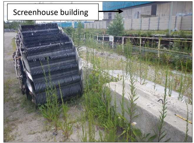
Photograph 87. DTE - Monroe Plant DSCN0173.JPG Description: Traveling screen next to the channel on the north side of the screen house building.
