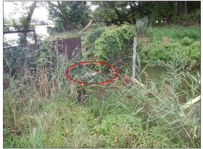
Photograph 63. DTE - Monroe Plant DSCN0149.JPG Description: View, facing southeast, of the Outfall 001F staff gage and effluent sampling weir (circled).
