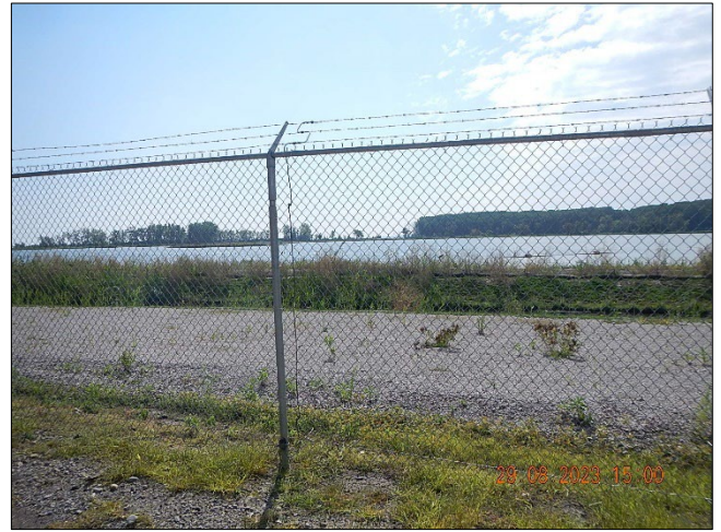
Photograph 27. DTE - Monroe Plant DSCN0113.JPG Description: View, facing west, of the inactive bottom ash basins and south process pond.
