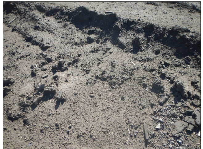
Photograph 72. DTE – Monroe Plant DSCN0158.JPG Description: The CCR Vertical Extension is used to dispose of bottom ash. Close view of bottom ash at the CCR Vertical Extension.
