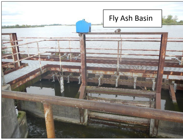
Photograph 57. DTE - Monroe Plant DSCN0143.JPG Description: General view looking west across the Fly Ash Basin from the Box Weirs Discharge Control Structure.
