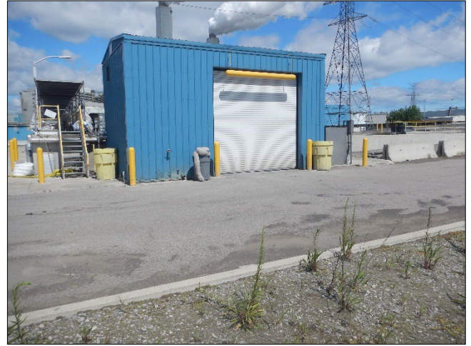
Photograph 115. DTE - Monroe Plant DSCN0201.JPG Description: View of the equipment shed and spill kits on the west side of the Bottom Ash Transfer Area sedimentation basins.
