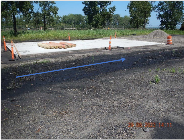
Photograph 9. DTE - Monroe Plant DSCN0095.JPG Description: View, facing north, of ditch that receives discharge from SS#6.
