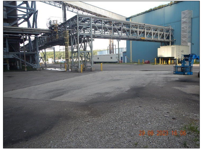
Photograph 43. DTE - Monroe Plant DSCN0129.JPG Description: General view of the generating building looking west from SS#3.
