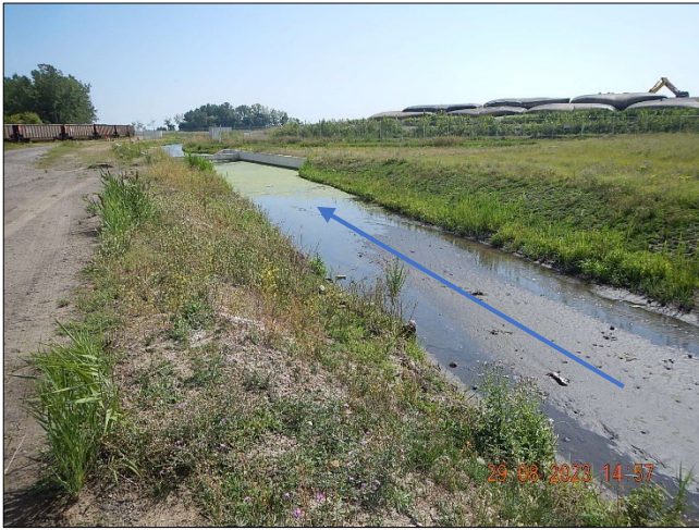
Photograph 25. DTE - Monroe Plant DSCN0111.JPG Description: View, facing southeast, of process swale channel.
