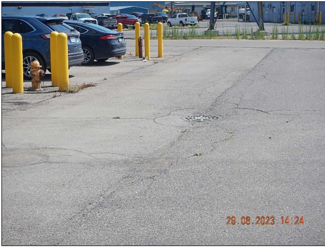
Photograph 17. DTE - Monroe Plant DSCN0103.JPG Description: General view of a drop inlet connected to SS#2.
