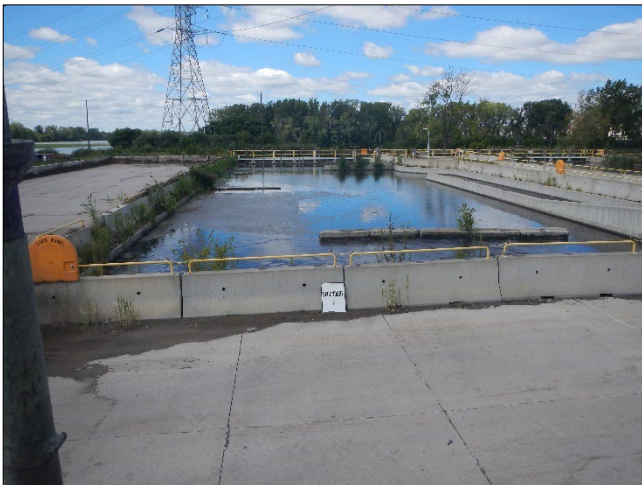
Photograph 110. DTE - Monroe Plant DSCN0196.JPG Description: View, facing west, of the Bottom Ash Transfer Area sedimentation basins.
