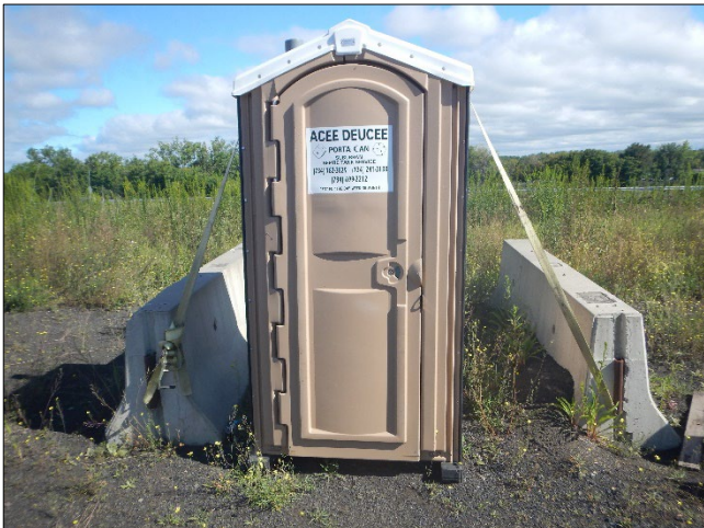
Photograph 78. DTE - Monroe Plant DSCN0164.JPG Description: The portable toilet at the CCR Vertical Extension equipment staging area was secured to the ground with tiedowns and stakes.
