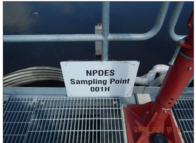
Photograph 32. DTE - Monroe Plant DSCN0118.JPG Description: View of 001H facing east towards the south process pond.
