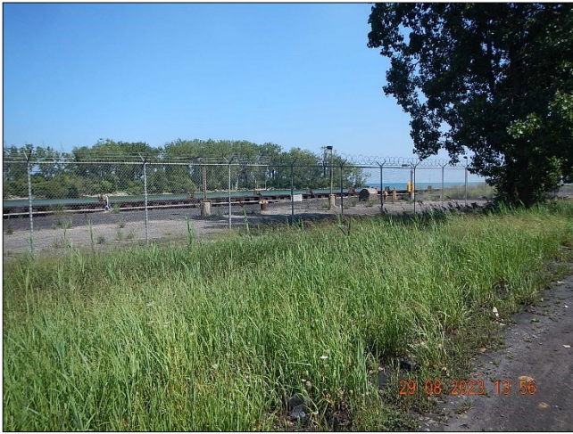
Photograph 5. DTE - Monroe Plant DSCN0091.JPG Description: View, facing northeast, of the dock on River Rasin next to the coal pile. The dock is beyond the fence line.
