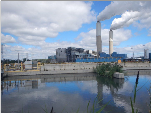
Photograph 114. DTE - Monroe Plant DSCN0200.JPG Description: General view of the Monroe Plant across the Bottom Ash Transfer Area sedimentation basins.
