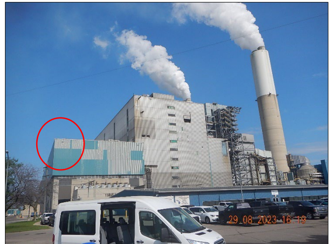
Photograph 48. DTE - Monroe Plant DSCN0134.JPG Description: View, looking northeast, at the Main Plant and PAC building in front of it. Roof drains on the northwestern side of the turbine house roof (circled) are piped to SS#1.
