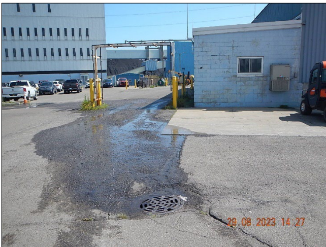
Photograph 18. DTE - Monroe Plant DSCN0104.JPG Description: View, facing north, of inlet below a vehicle wash station at the Motor Pool. The inlet connects to SS#2.
