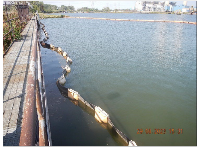
Photograph 39. DTE - Monroe Plant DSCN0125.JPG Description: View, facing north, of the walkway next to the inactive bottom ash basin.
