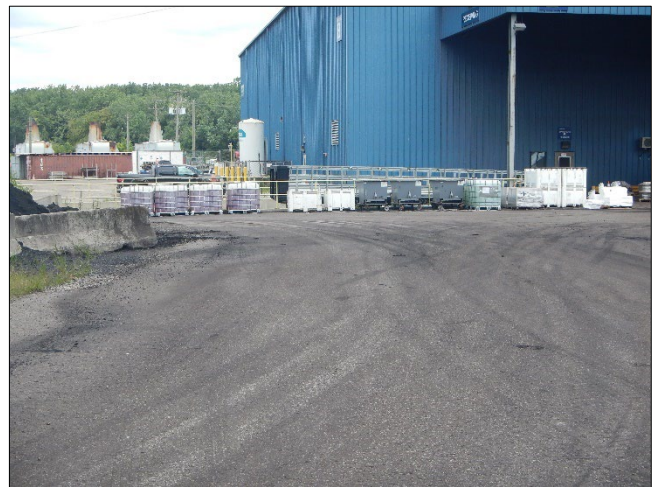
Photograph 92. DTE - Monroe Plant DSCN0178.JPG Description: View, facing north, of Warehouse B with totes and hoppers stored outside without cover or containment.
