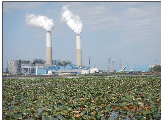
Photograph 28. DTE - Monroe Plant DSCN0114.JPG Description: General view, facing north, of the Monroe Power Plant.
