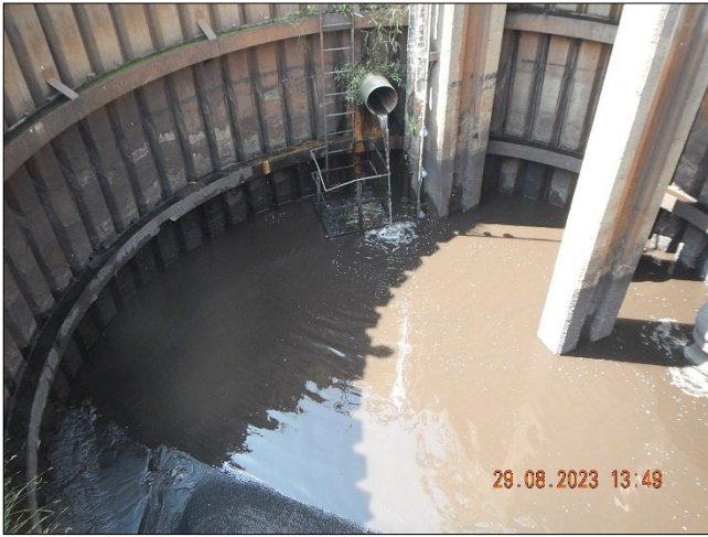
Photograph 1. DTE - Monroe Plant DSCN0087.JPG Description: View into Storm Station Number 6 (SS#6), by the coal pile handling area.
