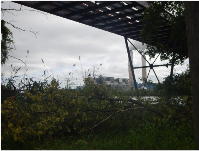
Photograph 69. DTE - Monroe Plant DSCN0155.JPG Description: View, facing east, at the Monroe Plant from underneath the four fly ash slurry lines that deliver fly ash from the Main Plant to the Fly Ash Basin.
