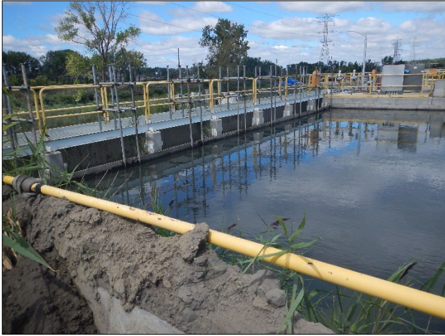
Photograph 113. DTE - Monroe Plant DSCN0199.JPG Description: View of the tail end of the Bottom Ash Transfer Area sedimentation basins.
