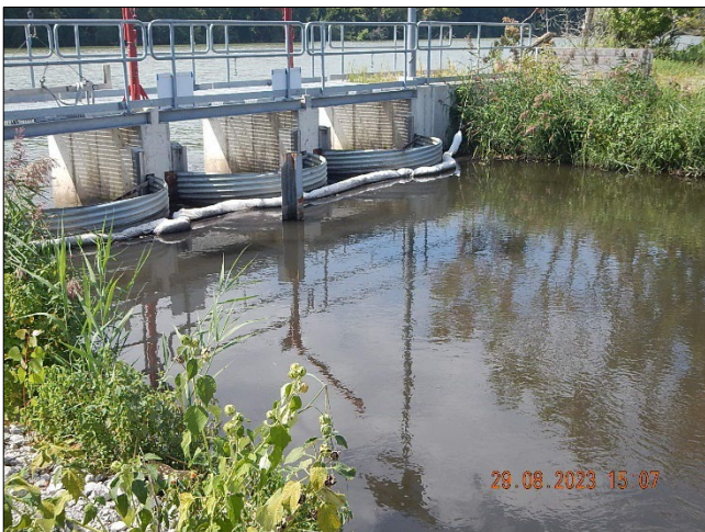
Photograph 30. DTE - Monroe Plant DSCN0116.JPG Description: View, facing west, of NPDES sampling station point 001H (001H) north of Outfall 001B from the south process pond side.
