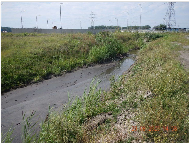
Photograph 26. DTE - Monroe Plant DSCN0112.JPG Description: View, facing northwest, of process swale channel.
