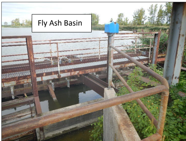
Photograph 58. DTE - Monroe Plant DSCN0144.JPG Description: General view looking northwest across the Fly Ash Basin from the Box Weirs Discharge Control Structure.
