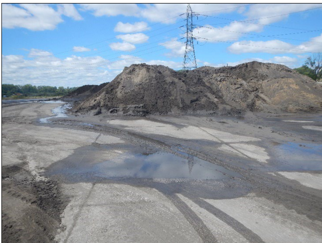
Photograph 106. DTE - Monroe Plant DSCN0192.JPG Description: View, facing south, of the Bottom Ash transfer Pad.
