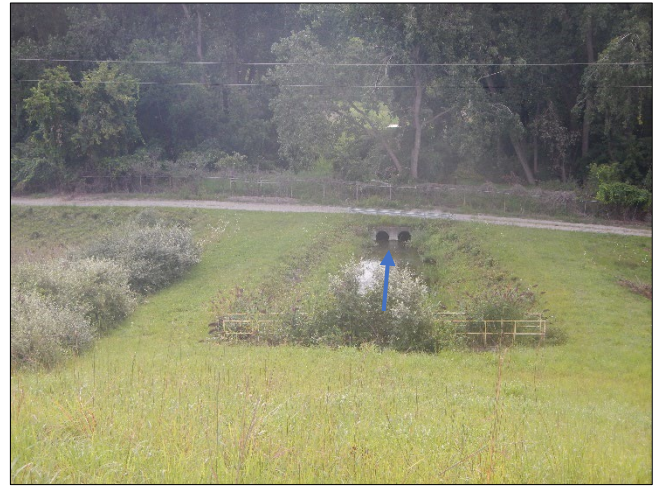
Photograph 55. DTE - Monroe Plant DSCN0141.JPG Description: View, facing east, at the channel between the Fly Ash Basin and Outfall 001F.
