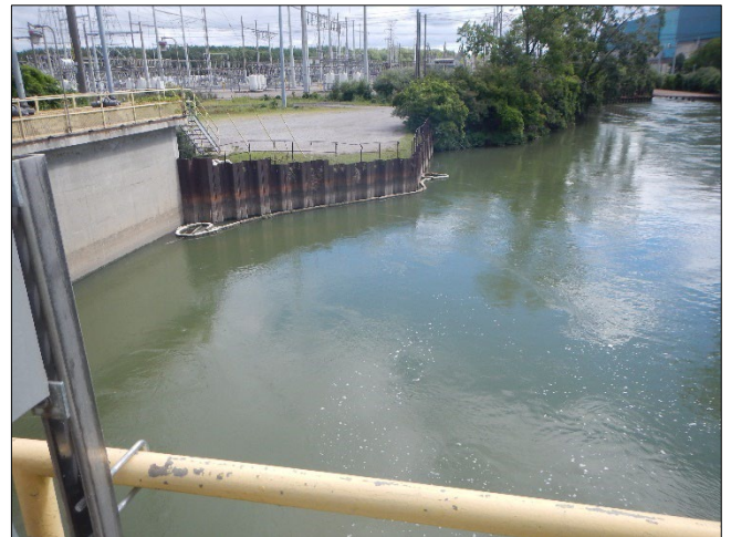
Photograph 84. DTE - Monroe Plant DSCN0170.JPG Description: General view, facing west, of the cooling water discharge canal from 001A. Booms (circled) were parallel to flow instead of perpendicular.
