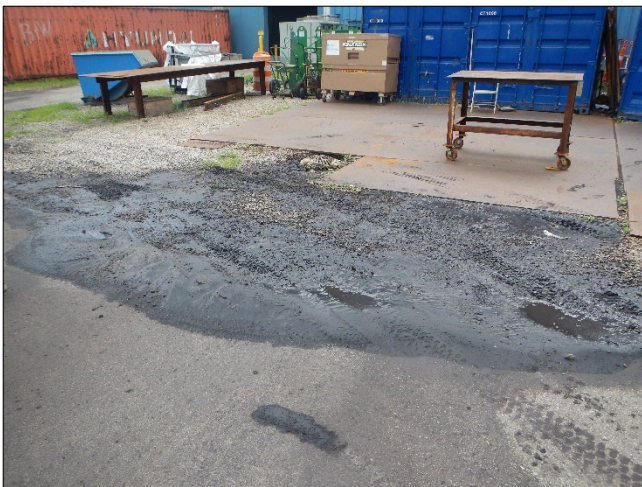
Photograph 90. DTE - Monroe Plant DSCN0176.JPG Description: Coal fines on the ground adjacent to the U2A Building. Runoff from this area goes to SS#4.
