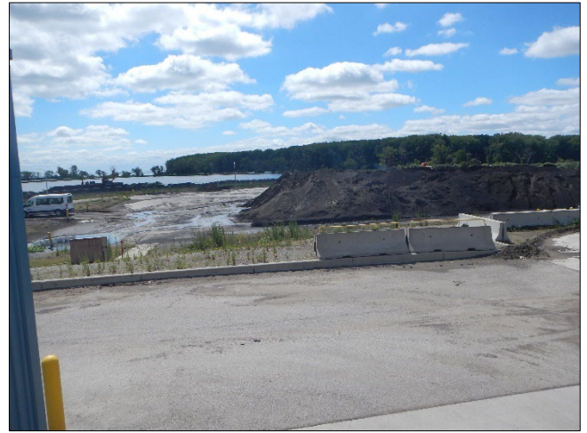
Photograph 111. DTE - Monroe Plant DSCN0197.JPG Description: View, facing south, of the CCR Transfer Pad and Bottom Ash Transfer Pad.
