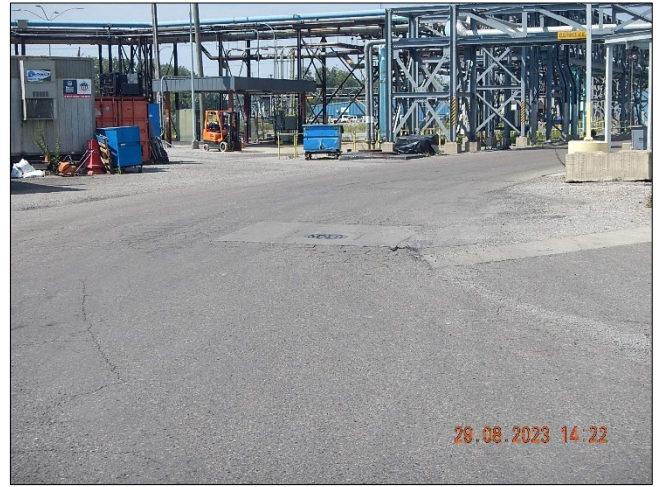
Photograph 15. DTE - Monroe Plant DSCN0101.JPG Description: View of a drop inlet located downgradient from the fueling area and the motor pool. This inlet connects to Storm Station (SS#2).
