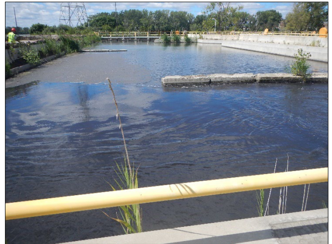
Photograph 112. DTE - Monroe Plant DSCN0198.JPG Description: Additional view, facing west, of the Bottom Ash Transfer Area sedimentation basins seen in Photograph 110.
