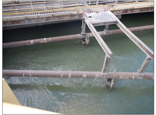
Photograph 83. DTE - Monroe Plant DSCN0169.JPG Description: View on the western side of the cooling water discharge canal. This area is directly after the location where samples were collected according to site representatives.
