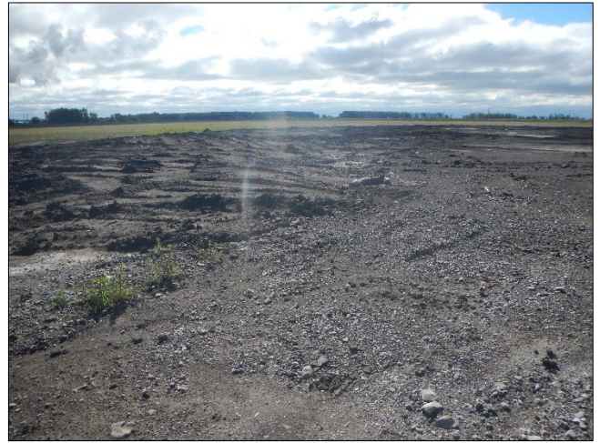
Photograph 71. DTE – Monroe Plant DSCN0157.JPG Description: View, facing southeast, across the CCR Vertical Extension. The CCR Vertical Extension is northwest of the Fly Ash Basin.
