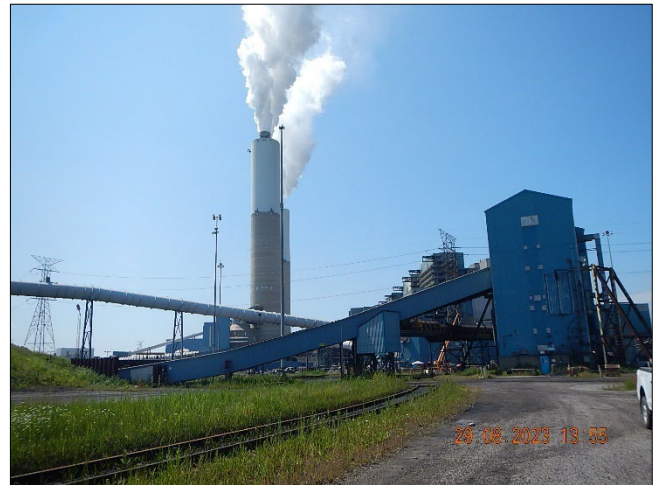
Photograph 4. DTE - Monroe Plant DSCN0090.JPG Description: Additional view of Main Plant seen in Photograph 3.
