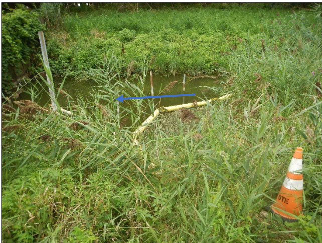
Photograph 62. DTE - Monroe Plant DSCN0148.JPG Description: View, facing south, of the channel between the Fly Ash Basin and Outfall 001F, just upstream of Outfall 001F.
