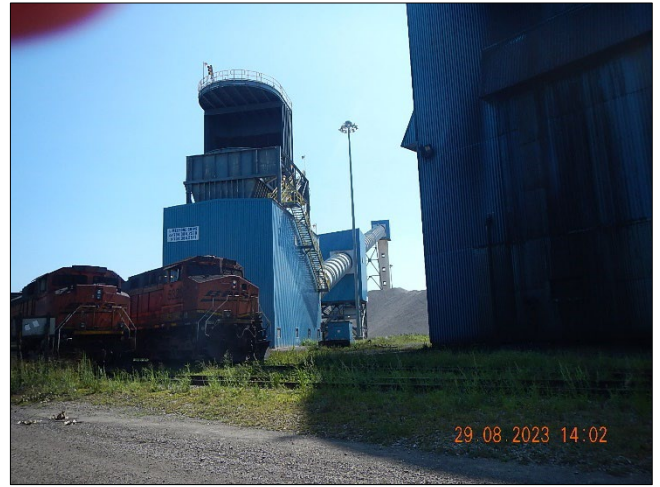
Photograph 7. DTE - Monroe Plant DSCN0093.JPG Description: Additional view of the coal transfer houses seen in Photograph 6.
