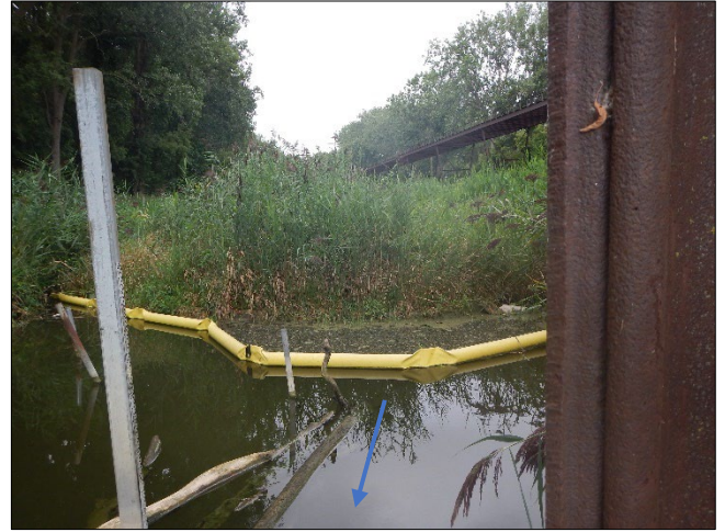
Photograph 67. DTE - Monroe Plant DSCN0153.JPG Description: View, facing west, from the Outfall 001F effluent sampling weir at the boom placed across the discharge channel to detain floatable material.
