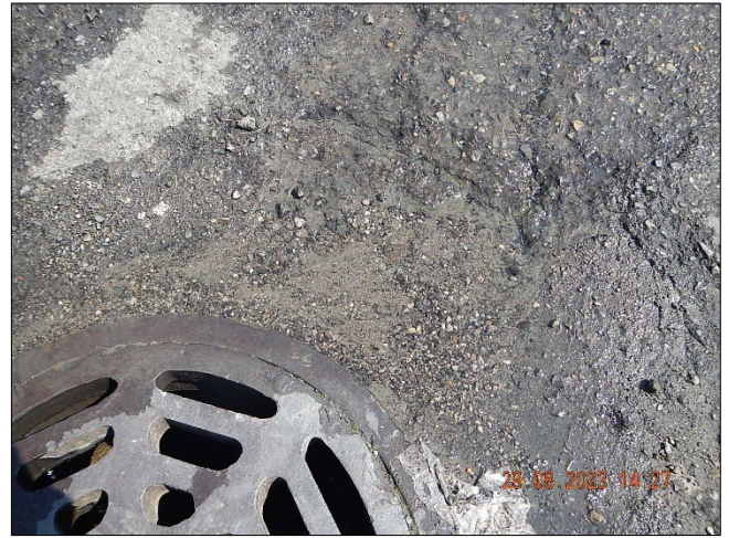
Photograph 19. DTE - Monroe Plant DSCN0105.JPG Description: Additional photo of the inlet seen in Photograph 18.
