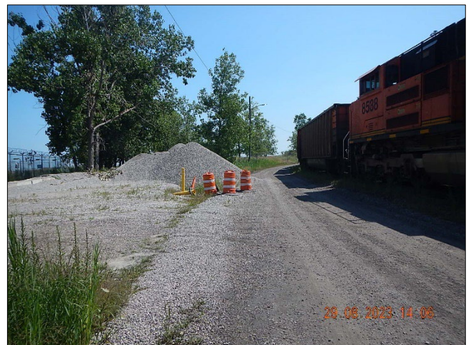
Photograph 8. DTE - Monroe Plant DSCN0094.JPG Description: View, facing east, of the road between the dock seen in Photograph 5 and coal transfer stations in Photograph 6 and 7.
