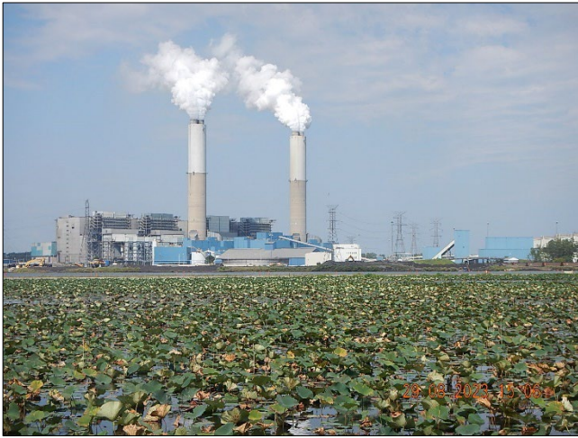
Photograph 29. DTE - Monroe Plant DSCN0115.JPG Description: General view, facing north, of the Monroe Power Plant.
