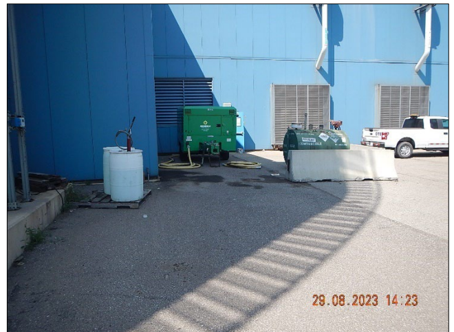
Photograph 16. DTE - Monroe Plant DSCN0102.JPG Description: View, facing north, of two 50-gallon barrels with diesel exhaust fluid (DEF) stored outside not undercover and without secondary containment. Also pictured are a portable generator and double-walled diesel tank.
