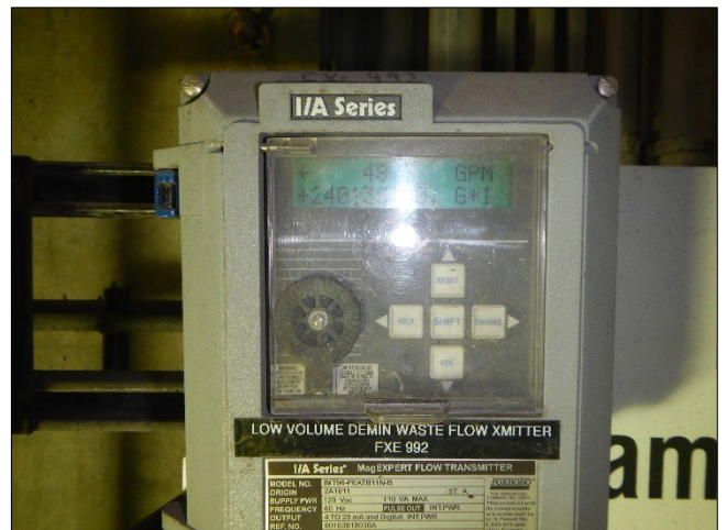
Photograph 104. DTE - Monroe Plant DSCN0190.JPG Description: Flow rate through NPDES Sampling Point 001D.
