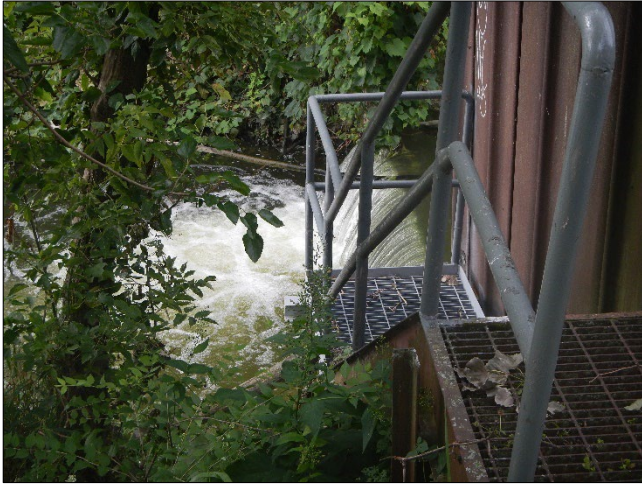
Photograph 65. DTE - Monroe Plant DSCN0151.JPG Description: View, facing south, of the downstream side of the Outfall 001F effluent weir.
