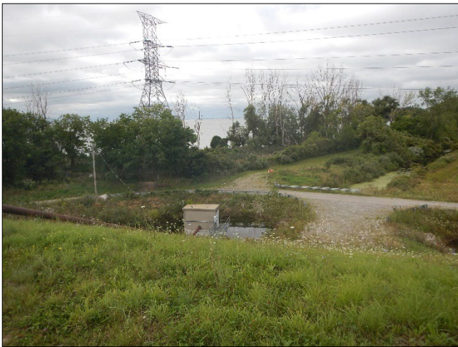
Photograph 54. DTE - Monroe Plant DSCN0140.JPG Description: Stormwater pump house at the southern corner of the Off-site Fly Ash Basin. The Off-site Fly Ash Basin is west and across the discharge canal from the Main Plant.
