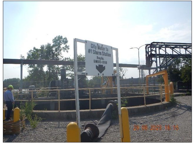
Photograph 47. DTE - Monroe Plant DSCN0133.JPG Description: View of SS#1.
