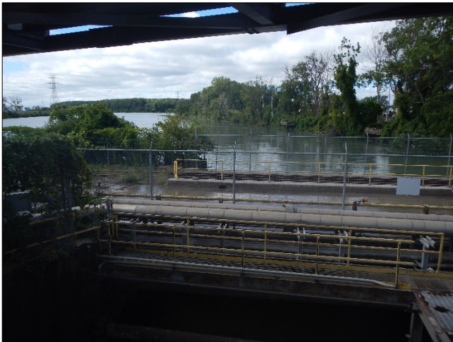
Photograph 82. DTE - Monroe Plant DSCN0168.JPG Description: General view, facing west, of where the discharge canal and cooling water discharge meet beyond 001A.
