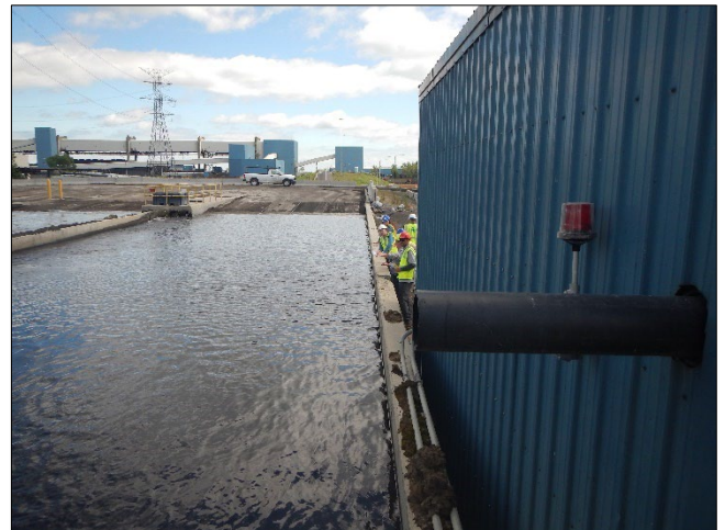
Photograph 108. DTE - Monroe Plant DSCN0194.JPG Description: View, facing east, of the Bottom Ash Transfer Area sedimentation basins.
