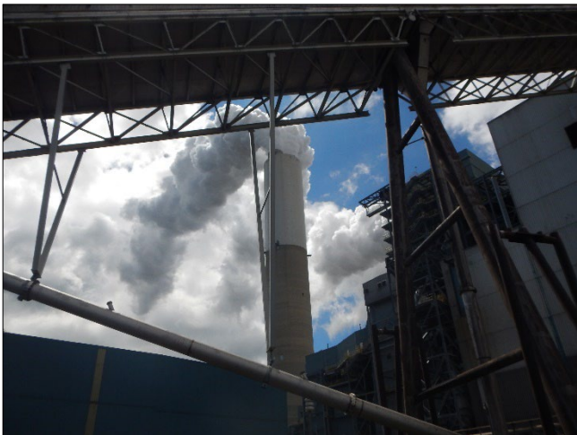
Photograph 98. DTE - Monroe Plant DSCN0184.JPG Description: Additional view of the Generating Building, as seen in Photograph 97.
