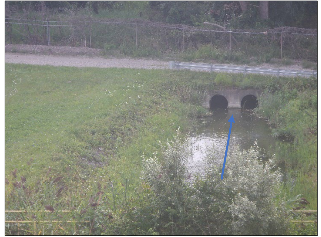
Photograph 56. DTE - Monroe Plant DSCN0142.JPG Description: Closer view looking east at the channel between the Fly Ash Basin and Outfall 001F.
