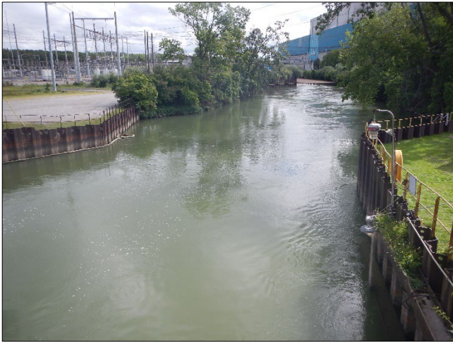
Photograph 81. DTE - Monroe Plant DSCN0167.JPG Description: View, facing east, at the cooling water discharge canal.
