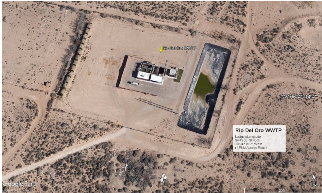
Aerial Image #1: Overall view of the Rio Del Oro Wastewater Treatment Plant. Aerial from Google Earth maps
