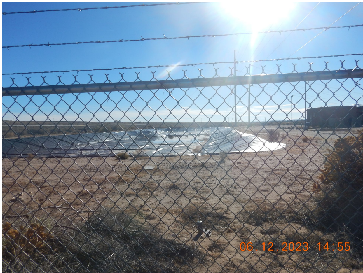
View looking south of the 500K-gallon emergency storage lagoon. (DSCN2675). Photographed by D. Esparza
