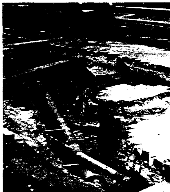
Installation of twin mail lines calked with lead, running under Barclay Street, New York, N. Y.
