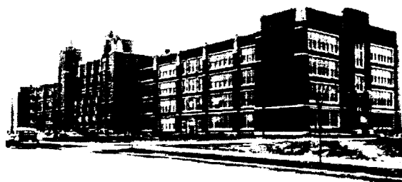
Mount Pleasant Regional Senior High School, Providence, R. I., where lead is used in the laboratory plumbing.
