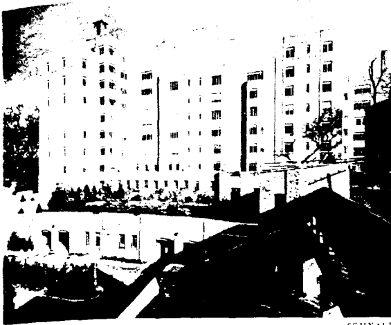
Full view of Hudson House, Ardsley-on-Hudson, N. Y. Shreve, Lamb and Harmon, architects.
