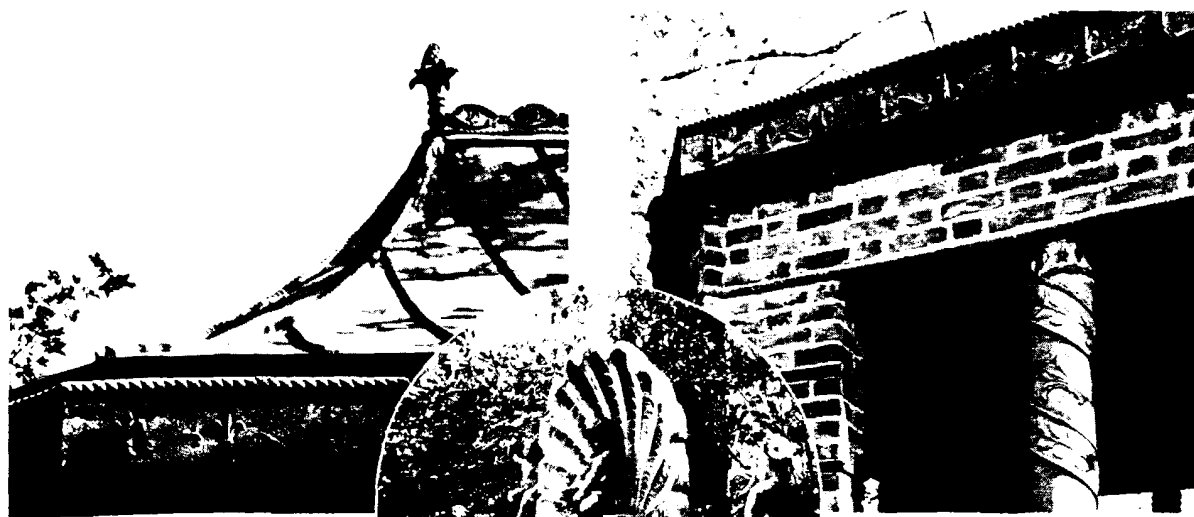
Close-up showing cast lead gutters, loose-locked, standing seam roof, ornamental rope molding, and lead crest and finial.
