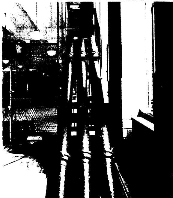
Pneumatic mail transportation lines in the new New York City Post Office Building, joined with lead as described in the article.
