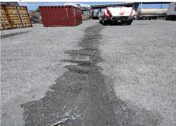
IMG 0111 -Evidence of stormwater runoff flow path from rear side of the maintenance shed, that runs across paved yard area.
