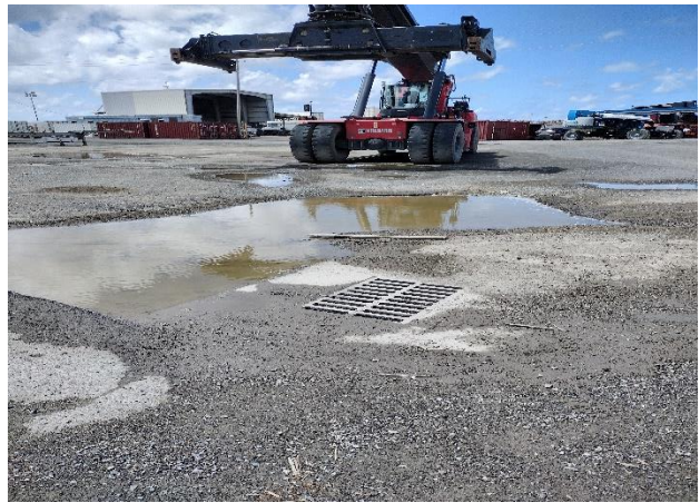
IMG 2816 -Retention area where stormwater runoff from the unpaved south section of CommUserArea 1 is collected and drained-off. Inlets are unprotected.
