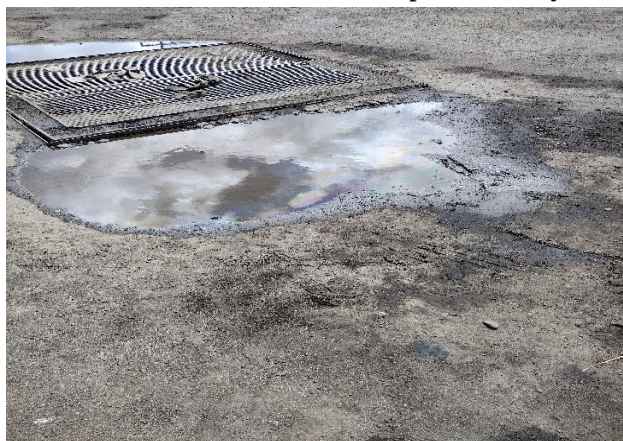
IMG 8118 -View of the large stormwater catch at low point in the yard of the maintenance shed. Oil spills patches next to the puddles observed.
