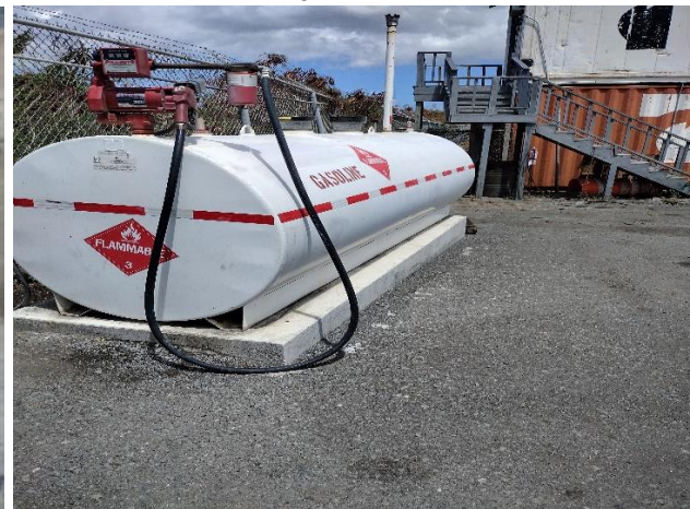
IMG 9911 -Closeup of fueling terminal unit with no containment around the system. Oil-soaked spot next to the tank, and exposed to stormwater runoff.
