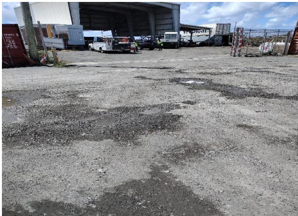
IMG 0179 -Sloped entrance into maintenance shed, where Tropical's vehicle fleet and equipment are regularly serviced. Potential for transport of sediments and gravel into stormwater catch basin.
