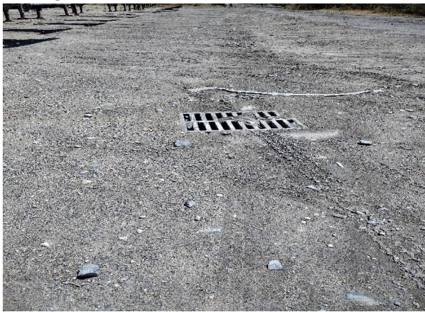
IMG 5058 -Partially clogged storm inlet midway of unpaved south section of CommUserArea 1.
