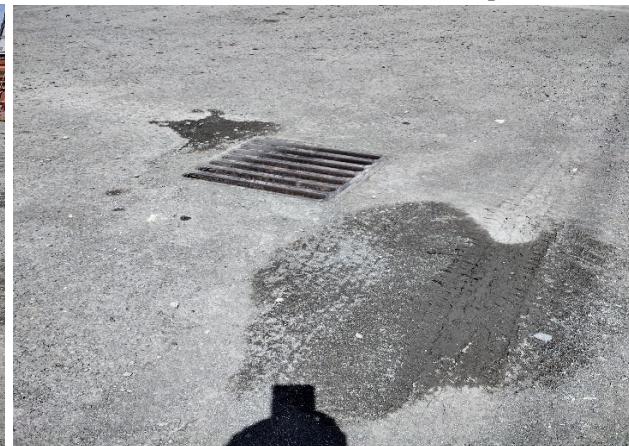
IMG 3660 -Accumulated sediment at base of sloped entrance into the Facility's maintenance shed area. Storm inlet unprotected from transport of sediment by stormwater runoff into stormwater catch basin.
