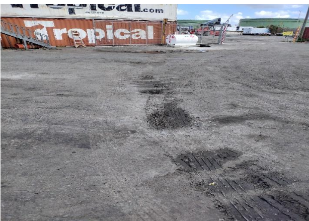
IMG 2768 -Close-up of stormwater runoff path that appeared saturated with oil patches along the stormwater path towards the stormwater catch basin.
