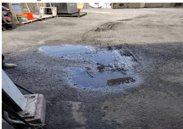
IMG 1616 -Stormwater runoff path observed from front of the shed flowing downhill towards a large stormwater catch basin at the low-point in the yard.
