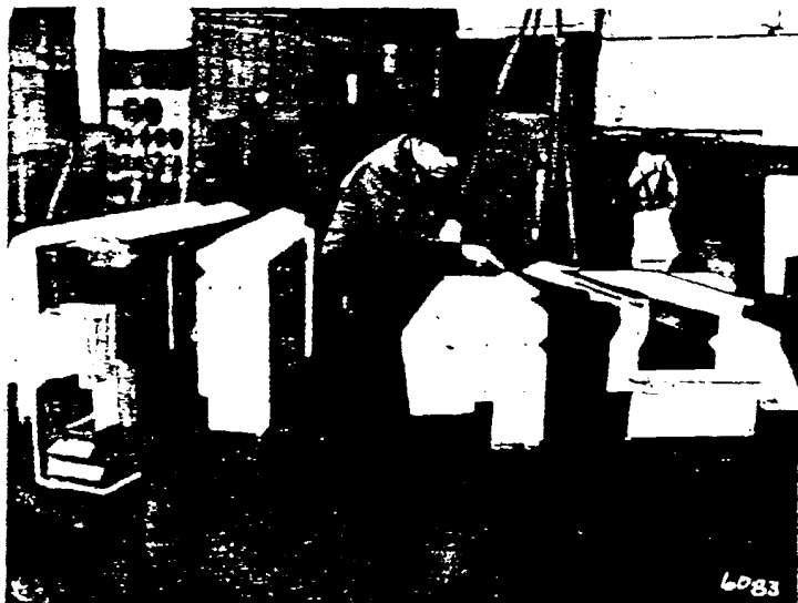
Below, component parts of lead shielding chambers. Lead is bonded to a 3-in. steel shell. Right, synchrotron before enclosure in outer casing, showing lead shielding in place.
