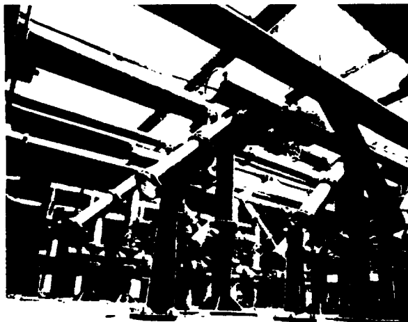
Inplant piping at New York City Newtown Creek Pollution Control Plant.
