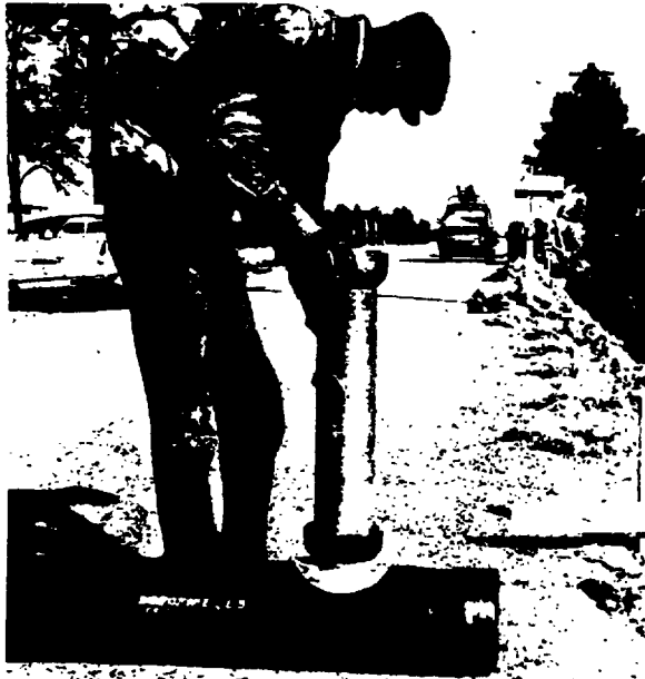
House sewer connection being set into 12-in. bituminized-fiber sewer pipe.
