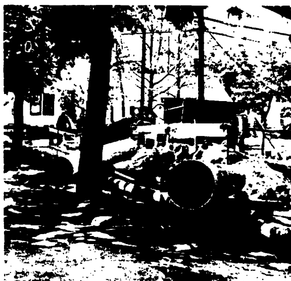
Well-point dewatering system along fully-sheeted trench for 24-in. asbestos-cement sewer pipe.
