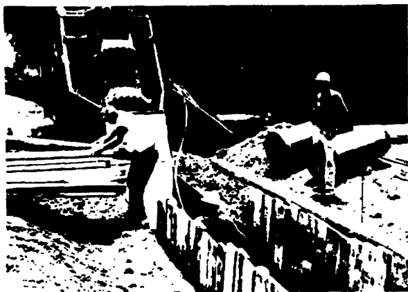
Large diameter, long length clay sewer pipe in fully sheeted trench.
