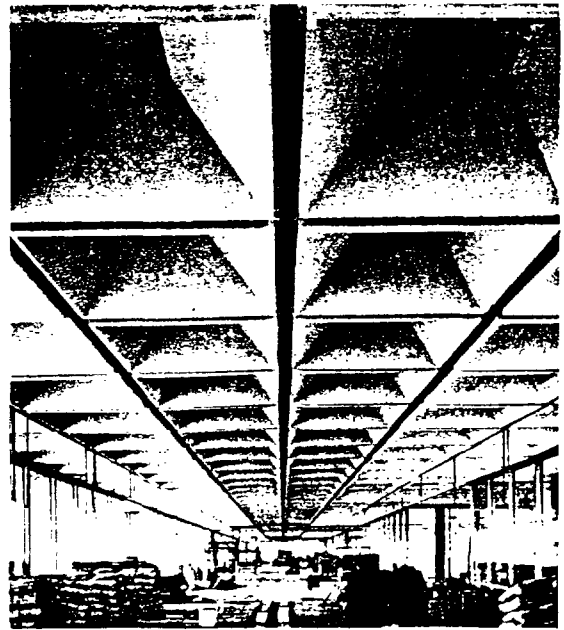
MORE THAN 4,000 pyramid-shaped plaster coffers cover spacious administration quarters of Upjohn Company's general office building. Coffers continue outside glass curtain walls.
