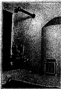
Therapy Room, St. Louis City Hospital, showing X-ray proof walls of barium sulphate plaster. Room in charge of Dr. L. R. Seale.
