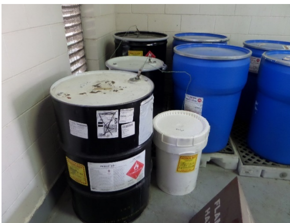
Picture 6: Lack of Aisle Space in Storage
